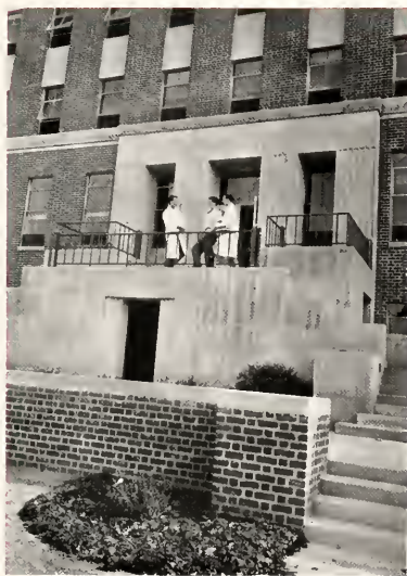
Front of the main building.
