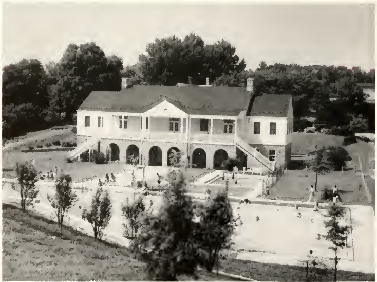
THE COMMUNITY HOUSE AND SWIMMING POOL
