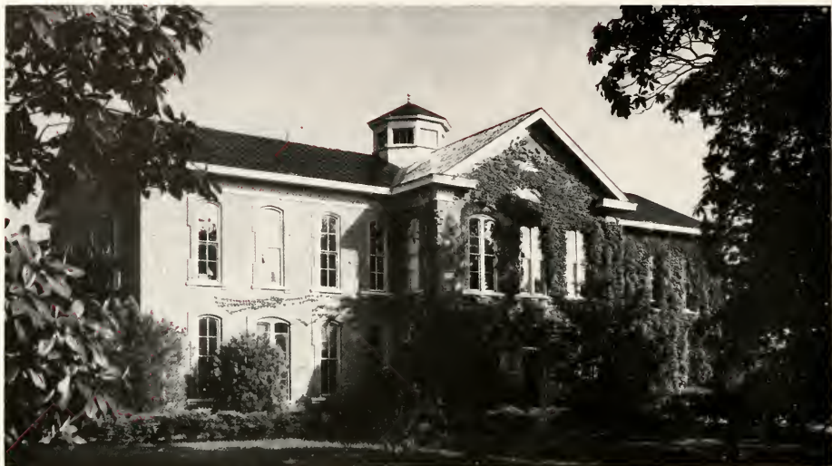
The Heck-Williams Library Building, home of the Law School
