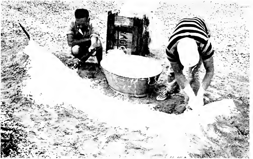
Fig. 175. The first or "splash" coat is applied. This step should be done in one uninterrupted operation.
