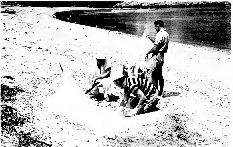
Fig. 176. The next coat of plaster is reinforced with sisal. Two assistants are required. In the field, local people usually are glad to help.
