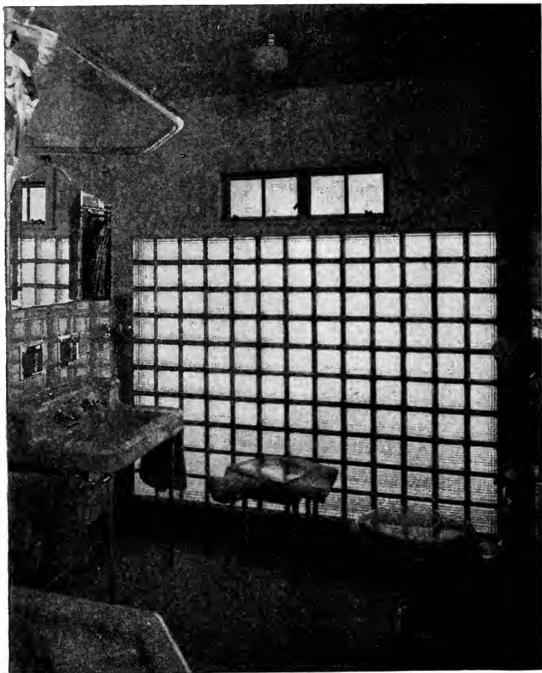
The picture above illustrates a very modern bathroom. The owner has made good use of the splendid possibilities of a glass block wall, but still provides ample ventilation through the two small high windows in the wall. (See Chapter IV.)
