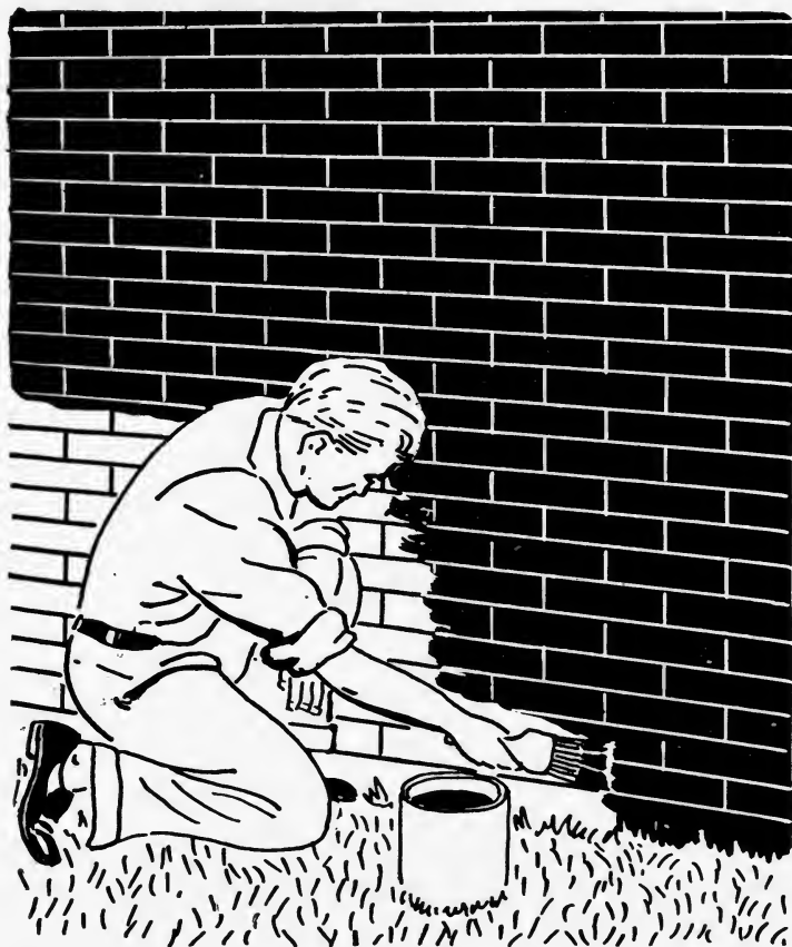
Porous or leaking brick walls may be tightened by the application of a good masonry waterproofing compound. Brick must be clean.
