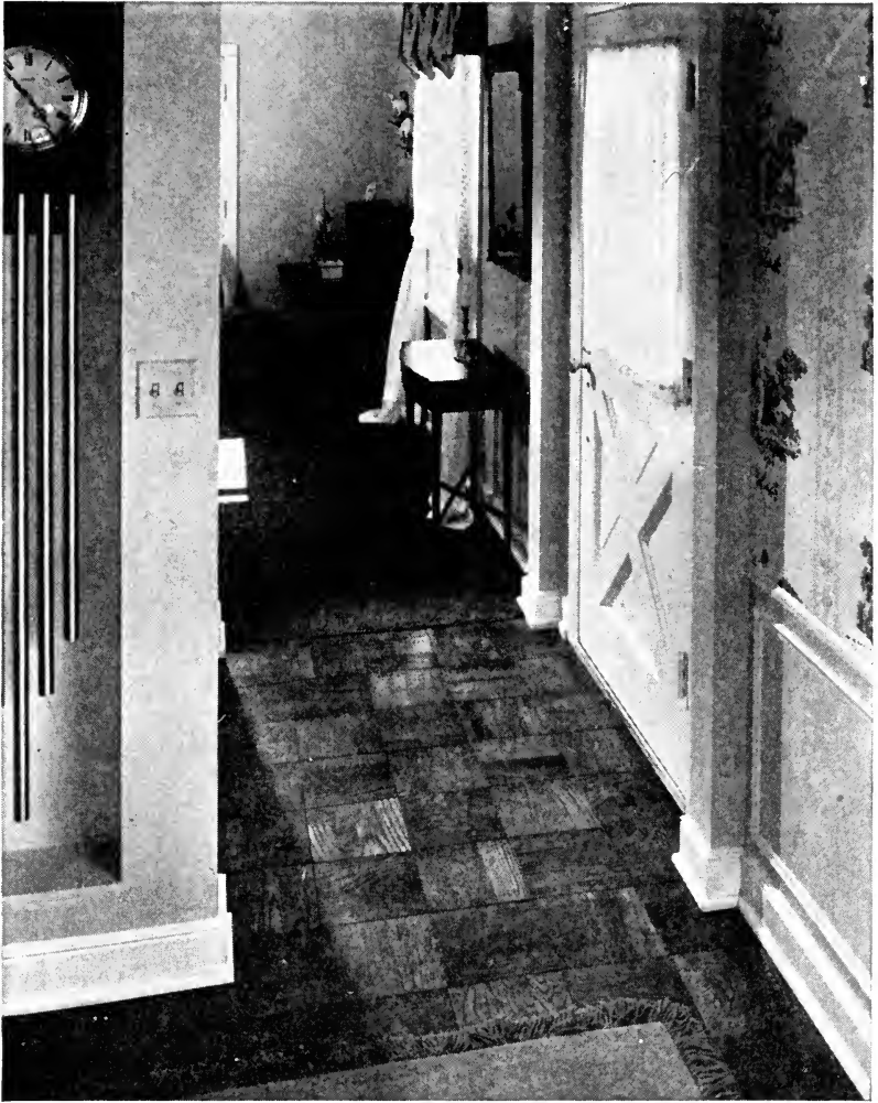
The treatment of floors depends entirely upon the worth of the floors. Certainly nobody would care to hide beneath a rug or carpets, the splendid inlaid hard-wood floor shown above. (See Chapter VIII.)
