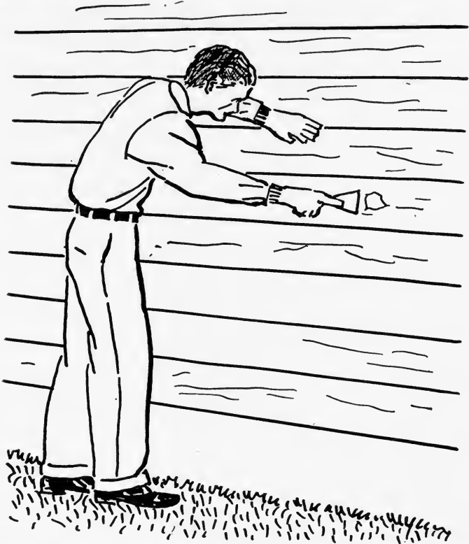
Painting over an unprepared surface is a waste of both time and materials. Loose paint must be removed and cracks filled.
