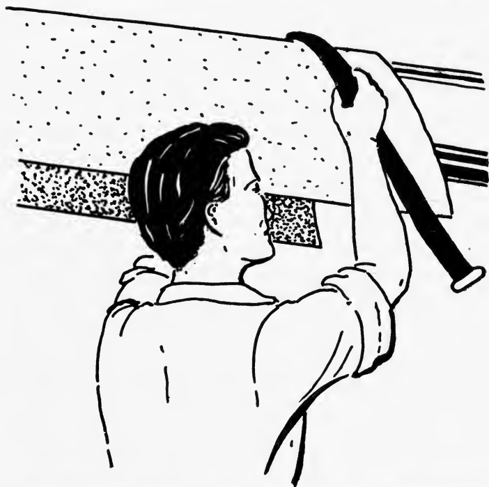
Asbestos-paper covering, will help to keep hot-air ducts from chilling. In cold cellars, this method has been highly effective.
