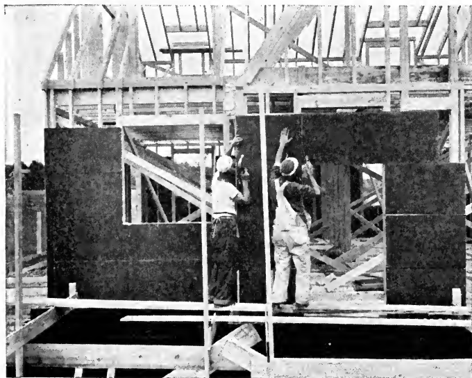
Beneath the exterior finish of the average house, there is a skin of material which backs up the outer wall. Wood sheathing has been a standard for many years. It is applied diagonally. Insulating board and plywood sheets have demonstrated their practical value in the small house building field. (See Chapter III.)
