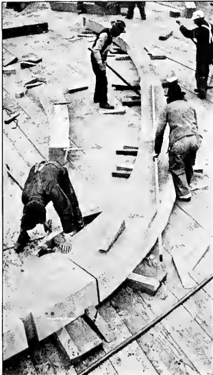
FIG. 51—ASSEMBLING FRAME PUTLOCKS ON FRAMING STAGE
