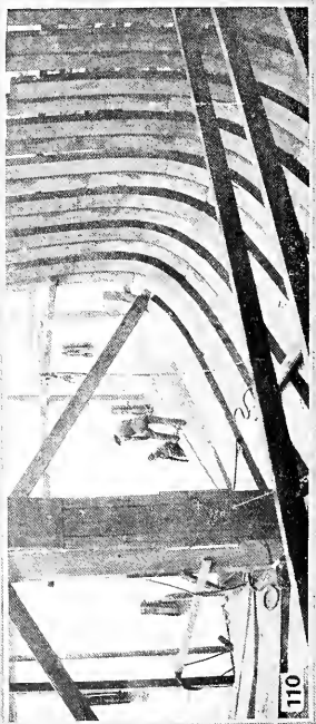
FIG. 106—DETAIL OF TRANSOM STERN FRAMING OF A SHIP UNDER CONSTRUCTION IN A SOUTHERN YARD. FIG. 107—TRANSOM TYPE STERN IN EARLY STAGES OF CONSTRUCTION. FIG. 108—THE NEXT STEP IN THE CONSTRUCTION OF A TRANSOM STERN. FIG. 109—INTERIOR OF A TRANSOM STERN BEFORE FASHION TIMBERS ARE IN PLACE. FIG. 110—A CLOSER VIEW OF THE INTERIOR OF THE SAME STERN. FIG. 111—FITTING TRANSOM TIMBERS TO FASHION TIMBER
