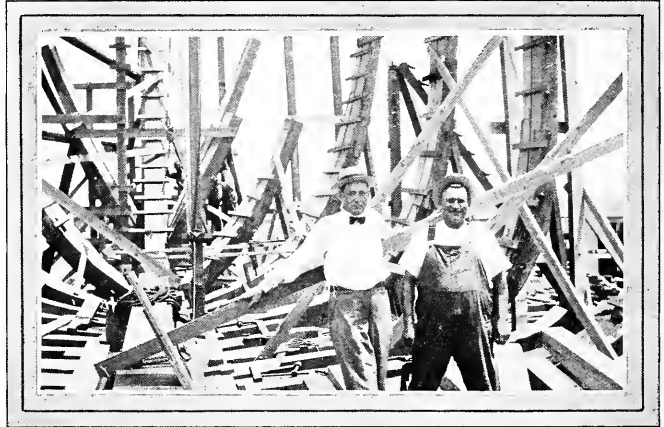
FIG. 99—DETAILS OF STEM AND FORWARD FRAME CONSTRUCTION OF A MOTOR SCHOONER UNDER CONSTRUCTION ON THE GULF
