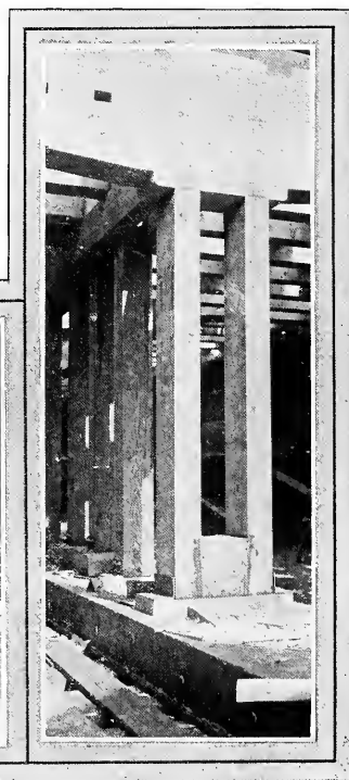
FIG. 154—DETAIL OF STANCHION FOOTINGS IN A LARGE WOODEN SHIP. FIG. 155—GENERAL VIEW OF STANCHIONS IN THE SAME SHIP
