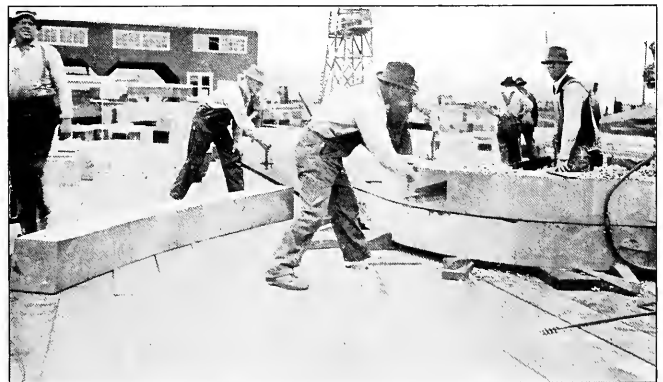
FIG. 52—RESAWING FRAME JOINTS TO A PROPER FIT
