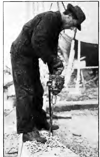
FIG. 11—BORING HOLES WITH AN AIR DRILL
