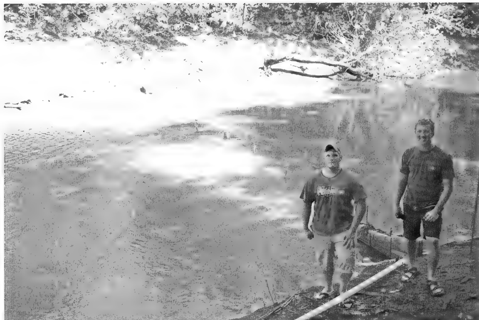
Anthony Erickson (left) and Blake Ruebush after installing a bubble barrier in Quiver Creek near Havana, Illinois. Photo by Michelle Horath, INHS
