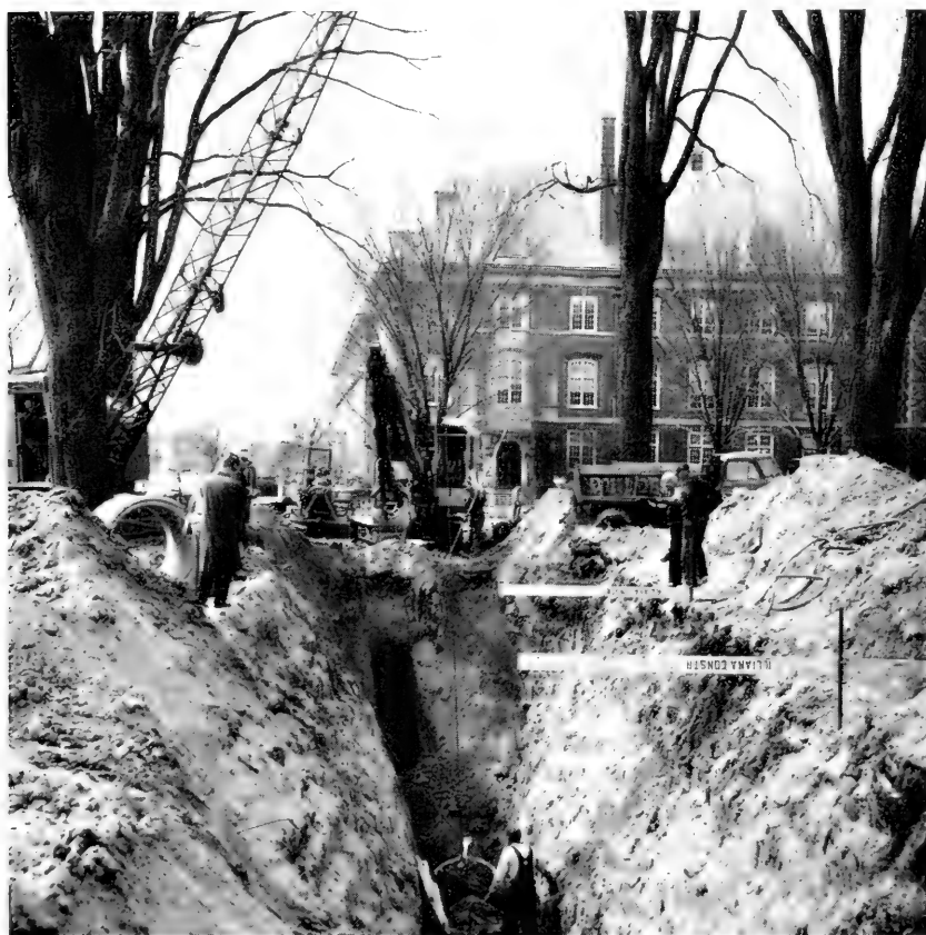
Fig. 6.—Yellowing and wilting of foliage on trees may be caused by root injury from excavation of soil. Such injury to elms may produce foliage symptoms similar to those of phloem necrosis. Mechanical injury of this kind may cause dieback of branches or death of trees.
