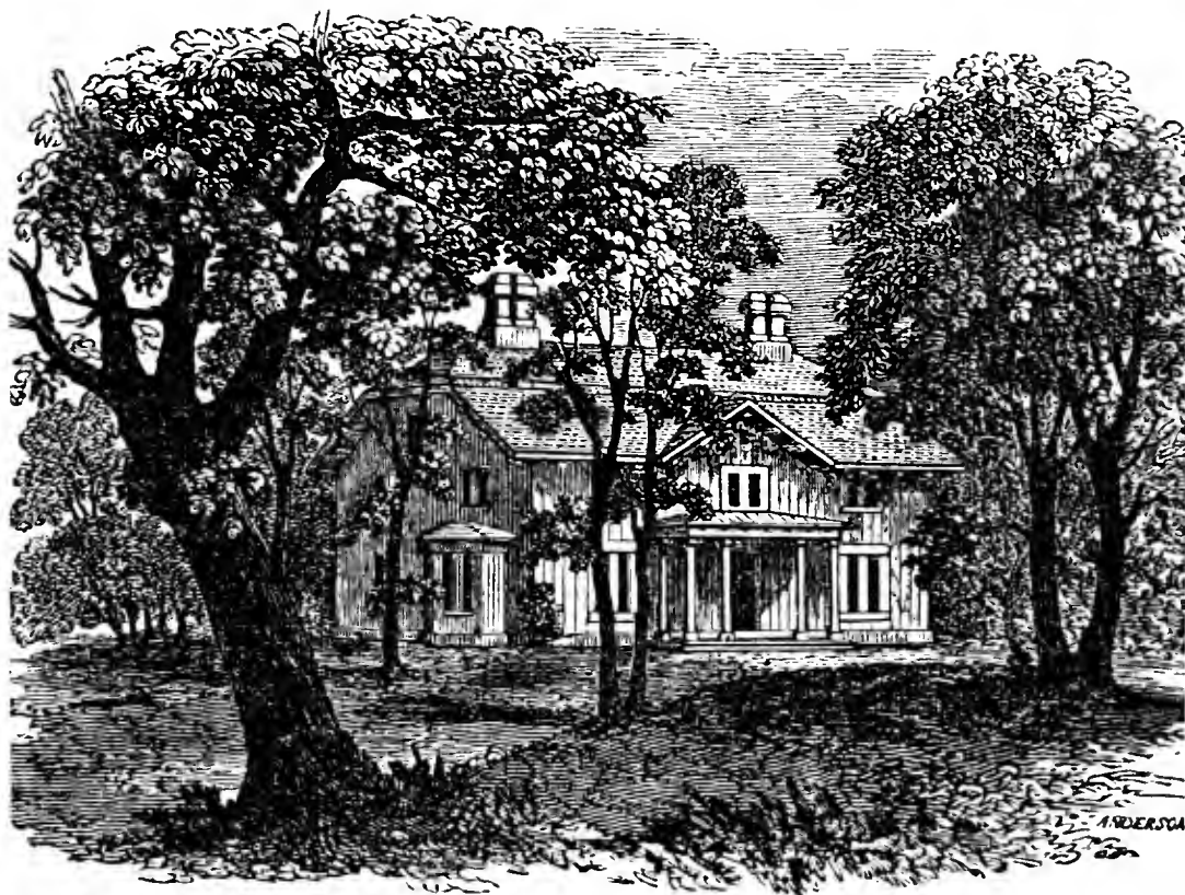
Fig. 54—BRACKETED FARM HOUSE.
