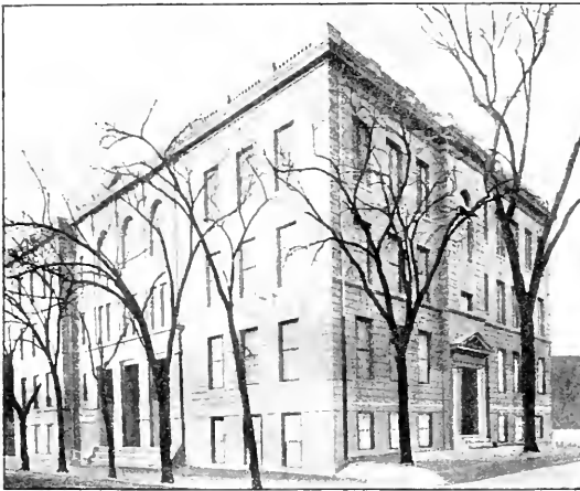
NEW BIGELOW SCHOOL, IN PROCESS OF CONSTRUCTION.
