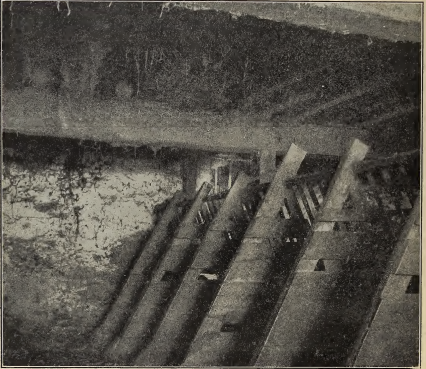
FIG. 3.—An undesirable stable. Note cobwebs heavily laden with dust, and wooden construction, which collects dirt and requires much labor to keep clean.
