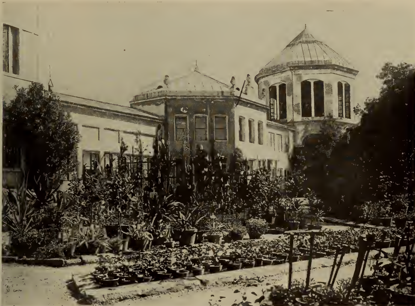
Building in Botanical Garden at Padua, showing rooms where Saccardo's herbarium is kept.
