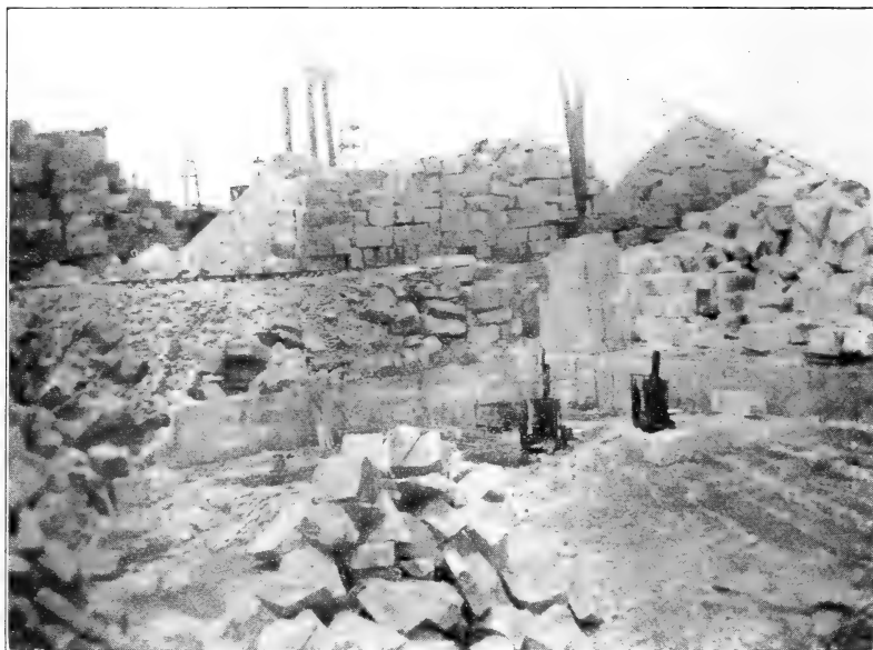
Looking northeast in the P. M. and B. quarry of the Indiana Quarries Company. This view shows how the storage of the waste stone often interferes with the quarry operations when the quarry is to be enlarged.
