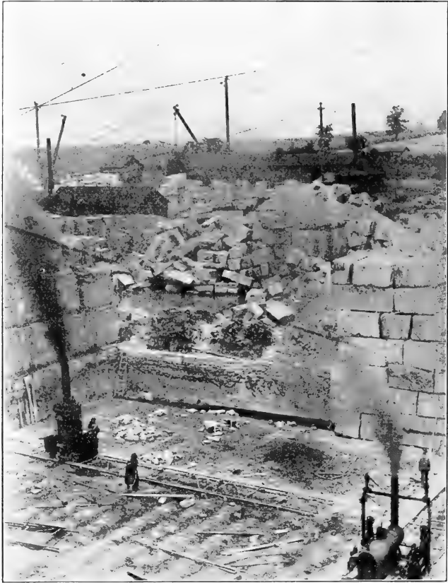
The waste piles of the National Stone Company's quarry at Clear Creek, Ind. In this case the waste has been stored well back out of the way of future operations.
