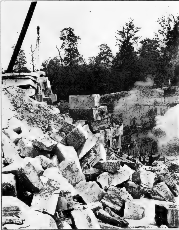
A corner in the quarry of the Crescent Stone Company at Hunter Valley, showing the method of waste disposal in use there.
