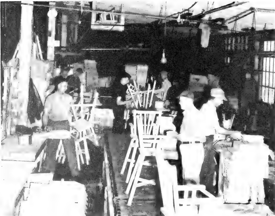
FIGURE 7.— This assembly line is turning out wooden high chairs—one of many products manufactured from wood in Indiana.
