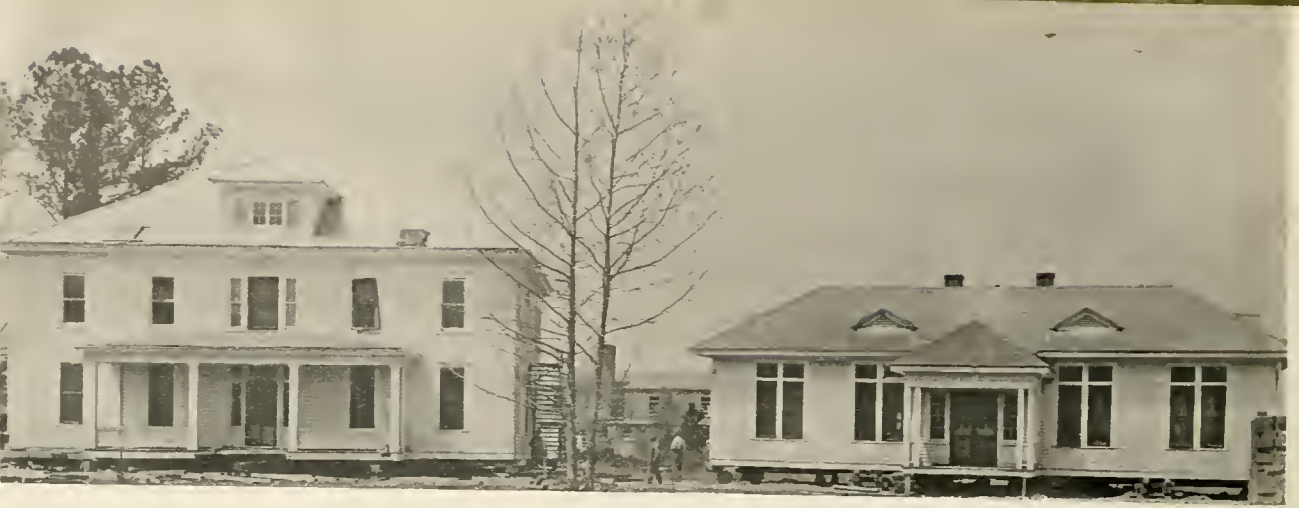
GIRLS' DORMITORY AND DINING HALL Being placed in present location
