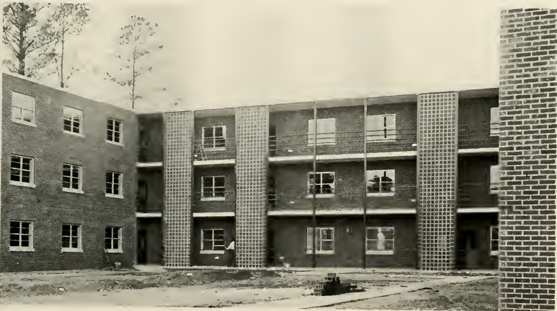
Construction of West Hall
