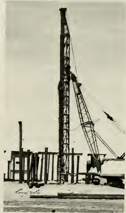
Construction on the new student center finally began in September 1985.
