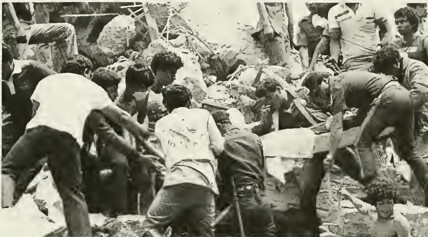
Rescuers dig hurriedly to find people buried under the collapsed hospital. Eight babies were found alive in that rubble.
