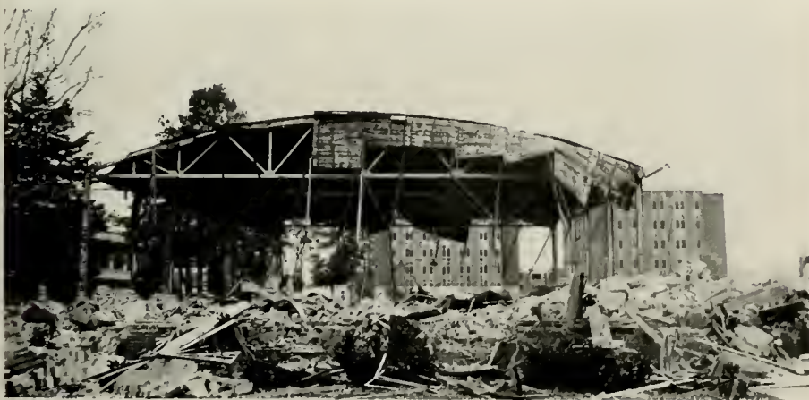
Old Gymnasium during demolition, October, 1988. Photo: Eric Smith.
