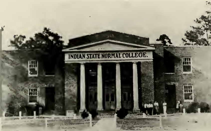
The face of Old Main, circa 1940. Like the institution, the structure has seen many changes.
