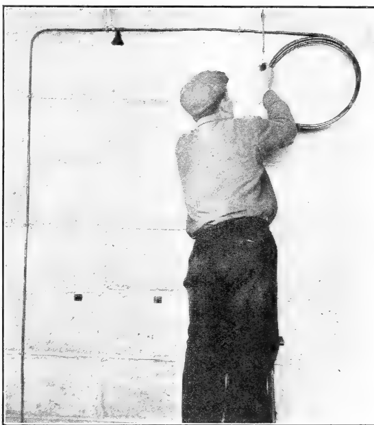
FIGURE 20.—Installation of three-eighths inch copper piping for introduction of liquid hydrocyanic acid. This piping, being flexible and easily cut with a saw, as indicated, can be run along side walls and out along rafters, or to any point where it seems best to install the spray nozzles.
