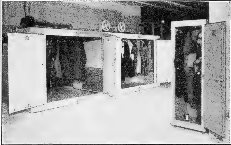
FIGURE 24.—Two types of metal vaults such as can be purchased or built according to space and commodity need. These vaults are used for treating the day's arrival of fur coats offered for summer storage. After an overnight fumigation in these vaults the furs are removed to large permanent storage vaults.
