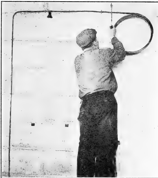
FIGURE 17.—Installation of \frac{3}{8} -inch copper piping for introduction of liquid hydrocyanic acid. This piping, being flexible and easily cut with a saw, as indicated, can be run along side walls and out along rafters, or to any point where it seems best to install the spray nozzles.
