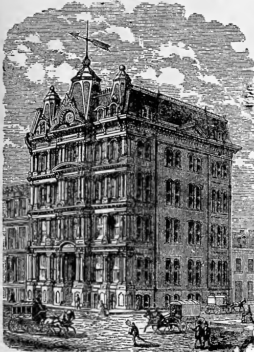
Germania Bank Building, cor. Wood St. and Diamond Alley.
