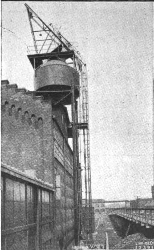
Link-Belt Skip Hoist, 103 foot travel, 25 tons per hour, at Iroquois Gas & Electric Co., Buffalo, New York.
