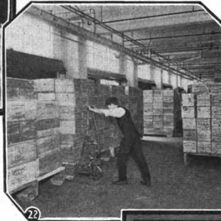
Fig. 22. In shipping rooms and warehouses, hand lift trucks are economical units. They facilitate easy and quick handling.
