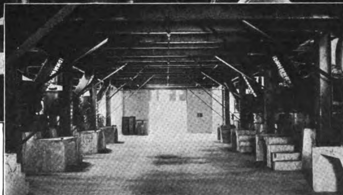
The larger installation shows top of coal mill and pipe connections to grinding mills, the trunk lines leading to Perfecto Filters as shown in illustration at top of this page. Dracco System improves the operation of any similar mill employing the air return principle.
