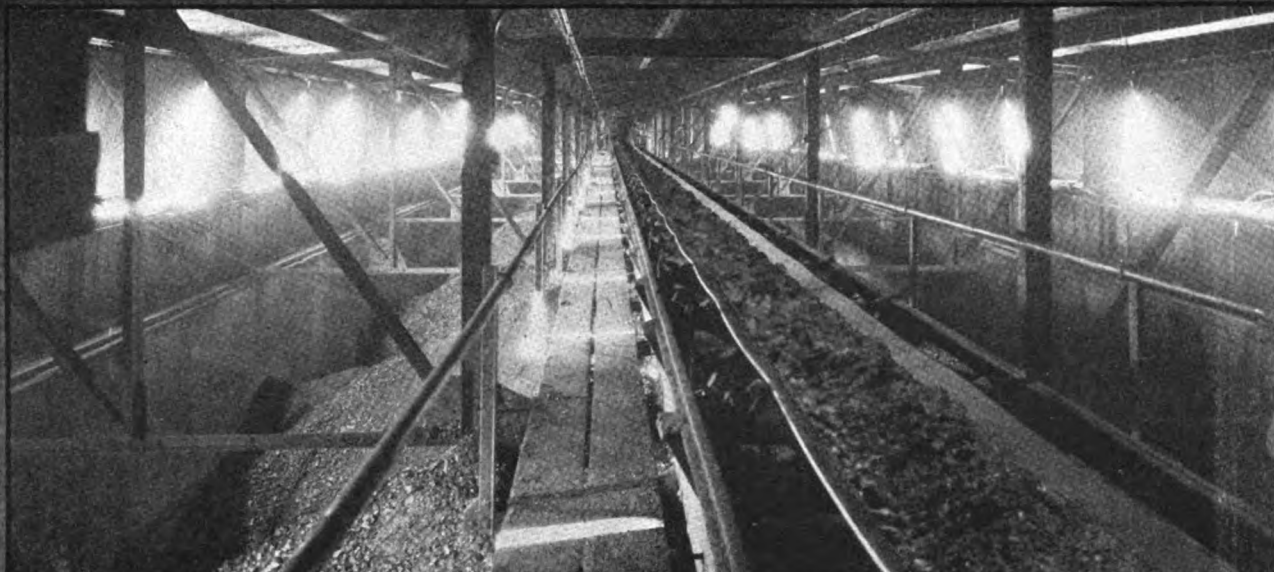
Belt Conveyor Distributing Coal to Overhead Bunkers
