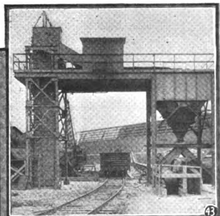
Fig. 43. A general view of the handling equipment for transporting new foundry sand from railroad cars to the various sand handling systems in the foundry.
