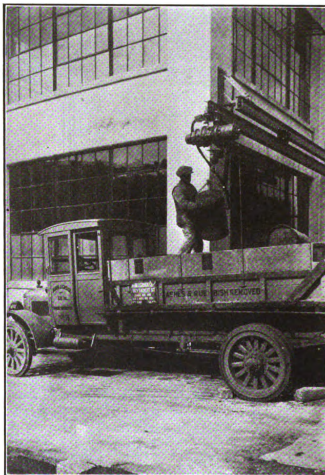
Fig. 22. Electric hoist and monorail trolley used for transporting and lifting ashes in cans.
