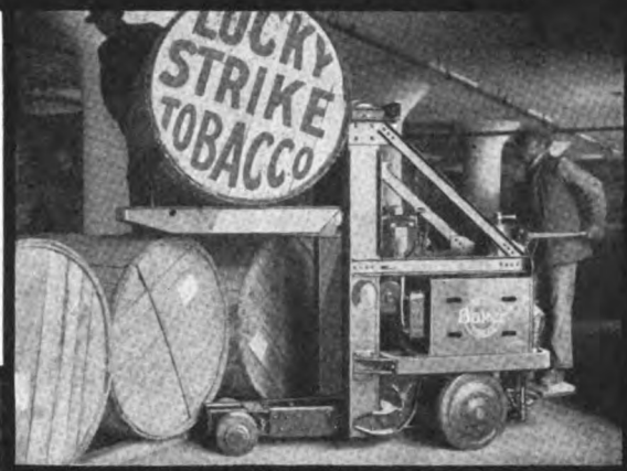
The Hy-Lift Truck lifts, carries and stacks heavy loads with ease.
