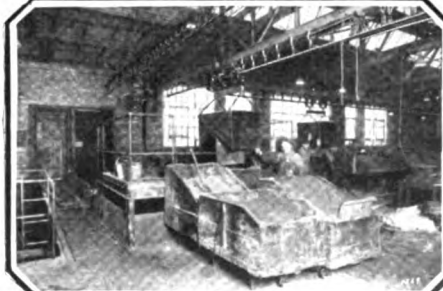
Reduced Pouring Gangs from 20 to 6 Men
