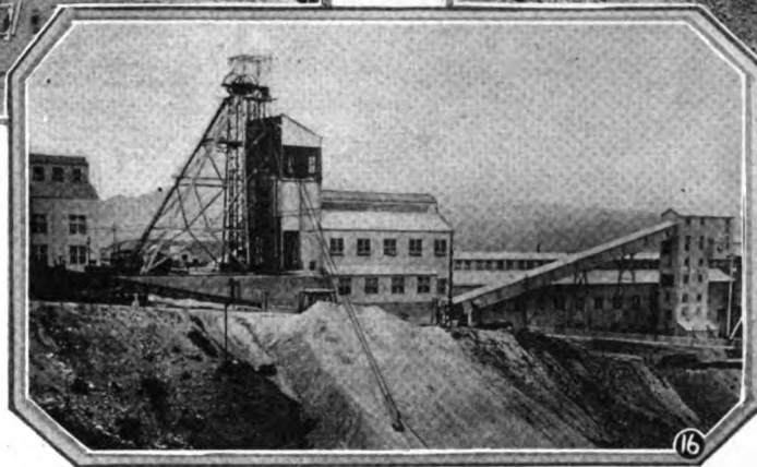
Fig. 16. Many industrial plants have found cableways of great assistance in handling materials on long hauls. This one is reclaiming copper tailing from hill-side dump and delivering same to car loading hopper at an Arizona refinery.
