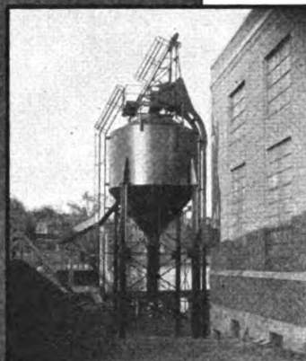
Ash Skip Hoist and Storage Bin
