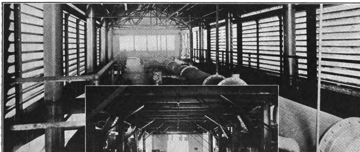
The larger installation shows top of coal mill and pipe connections to grinding mills, the trunk lines leading to Perfecto Filters as shown in illustration at top of this page. Dracco System improves the operation of any similar mill employing the air return principle.
