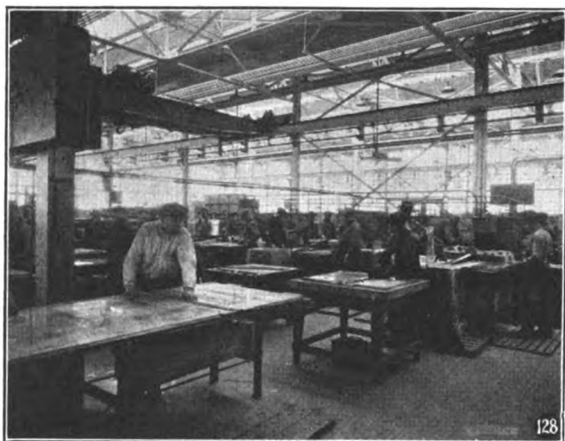
Fig. 128. General view of the glass cutting department, showing men cutting polished glass to the required sizes.
