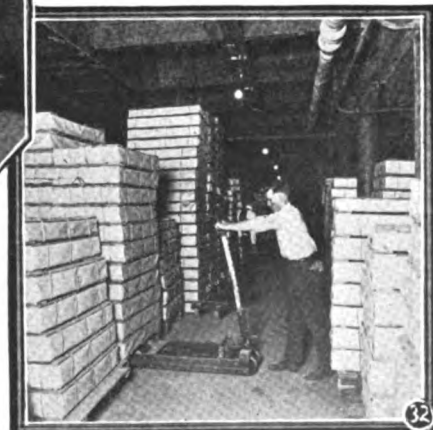
Fig. 32. Aisles should be at least as wide as the lift truck is long, preferably slightly wider. The necessity for this is clearly shown.
