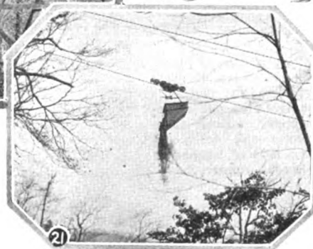
Fig. 19. Cableways are of great assistance on all new construction work. This shows such equipment operating on the construction of a new bridge.
