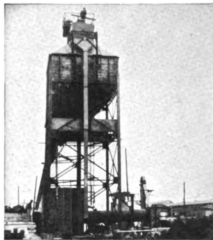
WELLER SAND HANDLING EQUIPMENT For Supplying Sand to Cars, Detroit Street Railway.
