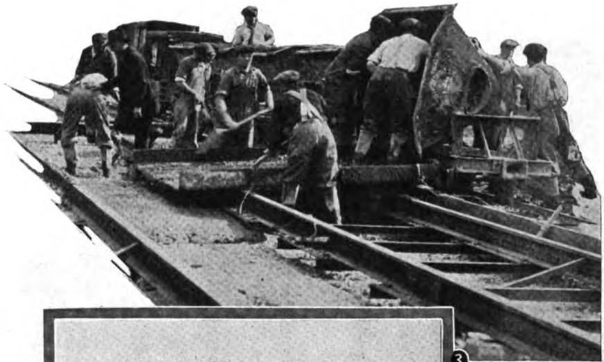
Fig. 3. Road builders are using this industrial materials handling equipment in the handling of concrete and they have found that it reduces their labor costs.
