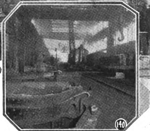
Fig. 140. The locomotive crane shown in this illustration is assisting in the installation of a new overhead traveling crane.
