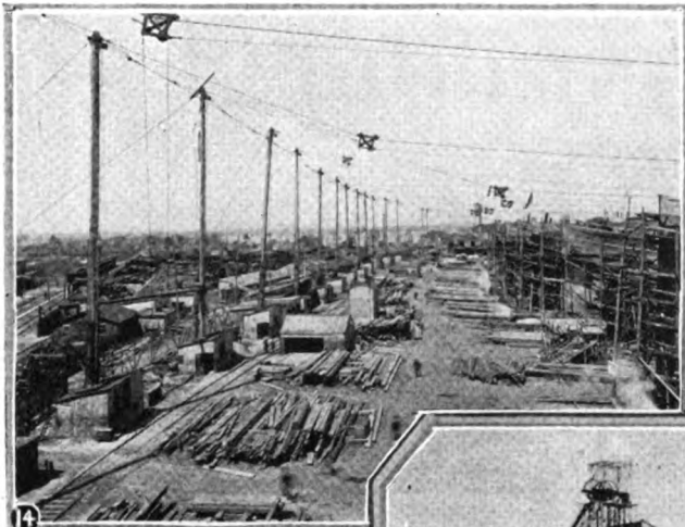
Fig. 14. This illustration shows a battery of fourteen cableways, used at the Portsmouth, New Hampshire, yards during the War. These cableways were so arranged that the masts at both ends could lean from side to side so that the cableways could reach any part of the ships on the ways.
