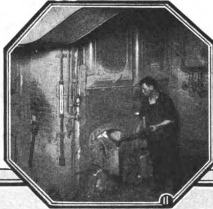
Fig. 11. CO 2 recorders are an important check on proper firing, and should be kept in condition by a competent man.
