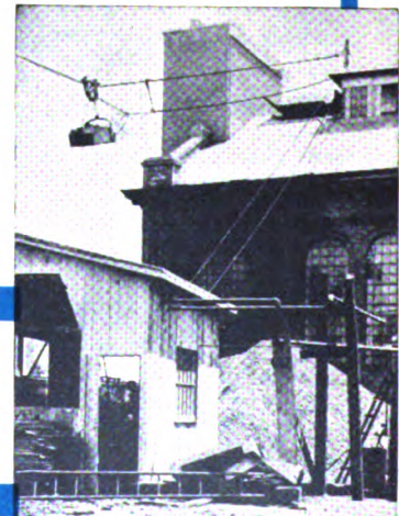
Cableway delivering material to top of plant structure
