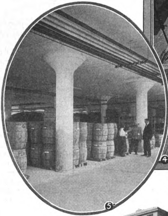
Fig. 5. A part of the storage cellar of the United Drug Company, St. Louis, Mo. The white cement finish makes for good lighting.
