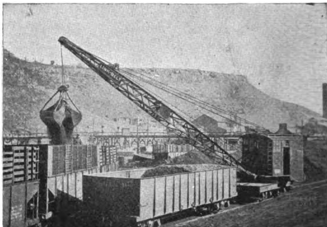
Link-Belt Locomotive Crane performs the service of from 20 to 40 men.
