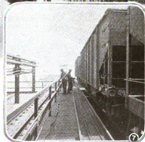
Fig. 7. Power driven cable hauls facilitate the movement of loaded and empty cars on high line.
