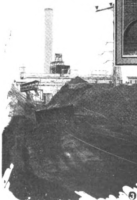
Fig. 3. Drag line scraper method of coal storage has been found efficient and economical.
