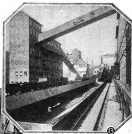
Fig. 13. A general view of some of the buildings and conveyor galleries which are shown in the diagrammatic view, Fig. 12.
