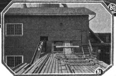
Fig. 80. General view of the saw mill, showing method of unloading logs and the conveyor elevating them to the gang saw.
