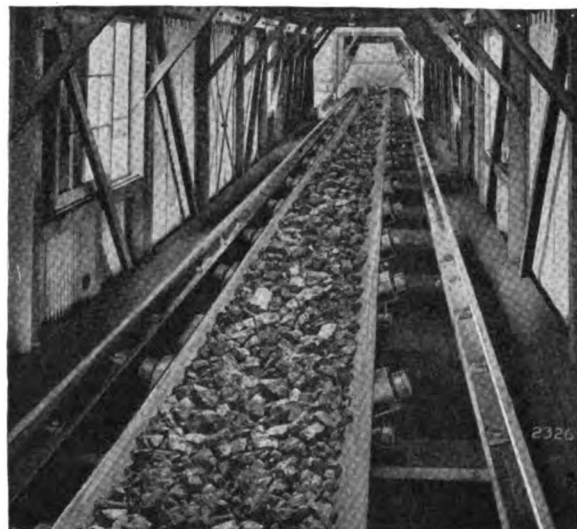
Link-Belt Belt Conveyor, one of the oldest known conveying devices.
