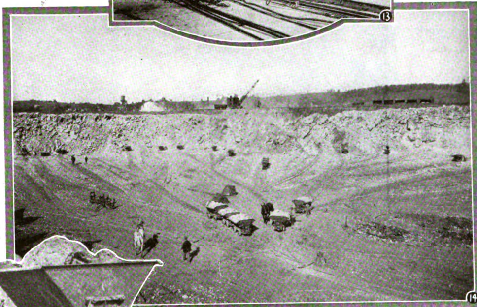
Fig. 14. Complete layout of track in limestone quarry where cars are loaded by hand.
