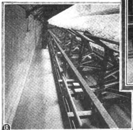
Fig. 18. A view in the coke wharf showing the method of feeding coke to the belt conveyor E, shown in Fig. 12.
