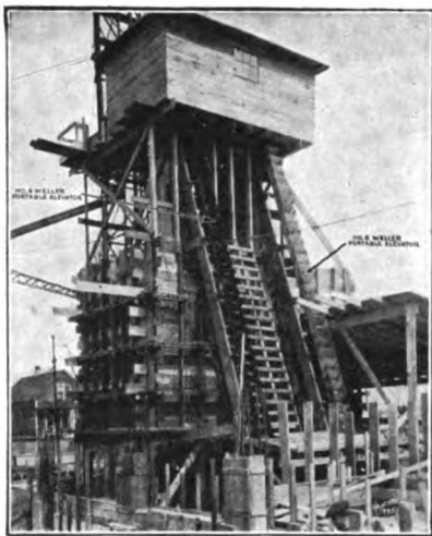
WELLER BUCKET ELEVATORS Used for Carrying Materials to Over-head Bins, Florsheim's Shoe Co.'s New Plant, Chicago.
