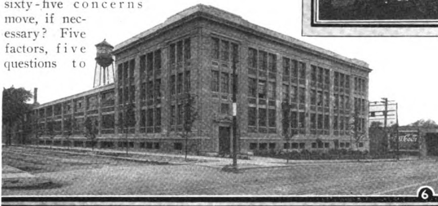
Fig. 6. One of the main plants of the Coca-Cola system. This is at Chicago.
