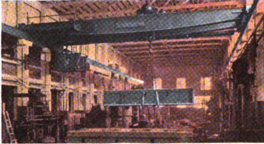
Electric Traveling Cranes
