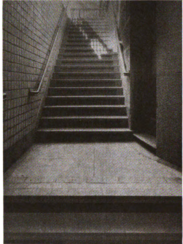
One of the latest subway installations of Norton Floors. Alundum Stair Tile on the steps of the Lawrence Street Station, Brooklyn-Manhattan Transit Corporation
