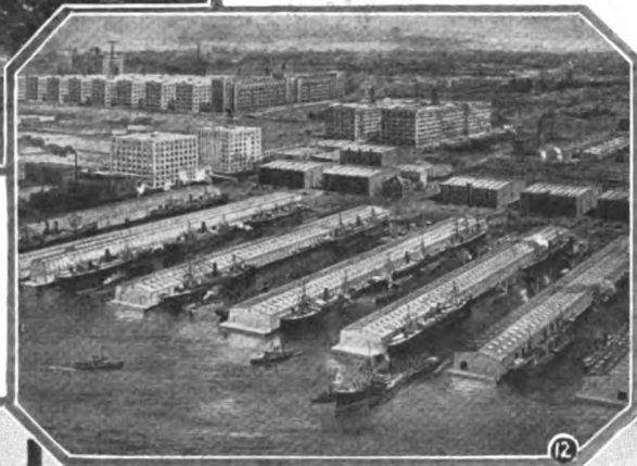
Fig. 12. The trend toward scientifically planned industrial areas is shown by the growth of the Bush Terminal, situated in Brooklyn on New York Harbor. Here large-scale planning and operation bring to several hundred concerns a combination of advantages impossible for the average individual concern.
