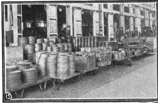
Fig. 16. For intra-plant transportation, or intra-building transportation, the loading of motor trucks with materials on lift platforms will save many handlings.
