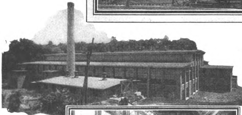
Fig. 13. Isolated plants, especially, require the carrying of spare parts to avoid costly delay in repairing breaks.
