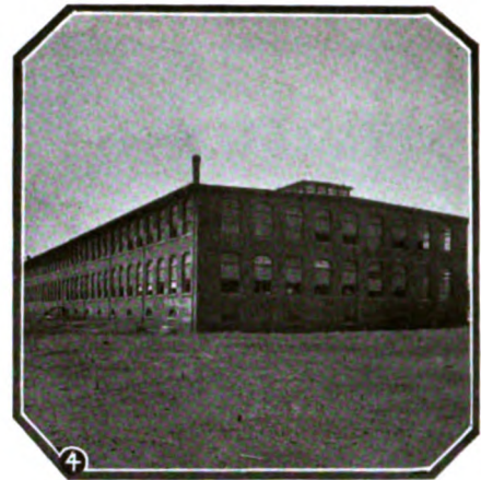
Fig. 4. The Union Bleaching and Finishing Cotton mill at Greenville, S. C., is near the cotton, has plenty of hydro-electric power, and can pay low wages because the workers enjoy low living costs. These are three of the reasons why the Southern textile industry is increasing rapidly.
