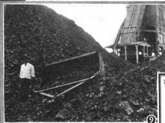
Fig. 9. A close-up view of the cable drag scraper handling run-of-mine coal in the actual installation of the equipment shown in Fig. 10.
