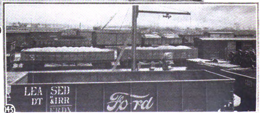
Fig. 145. This is a partial view of the miscellaneous freight yard at the north end of the plant, which is fully equipped with various mechanical handling devices.
