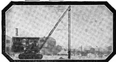
PILE DRIVING ATTACHMENT DRIVES ALL KINDS OF PILES.
