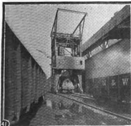
Fig. 41. Special gantry crane which pours hot metal from the ladle cars to smaller containers at the various hot metal spurs, shown in Fig. 33.
