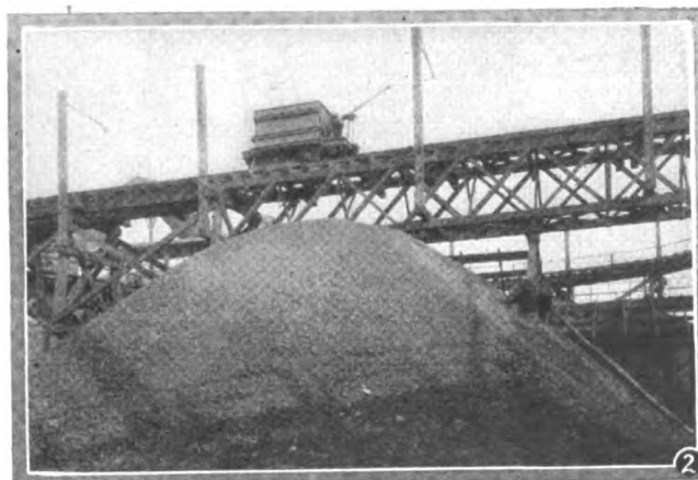
Fig. 2. Unit power driven car operating on trestle over outside storage yard.
