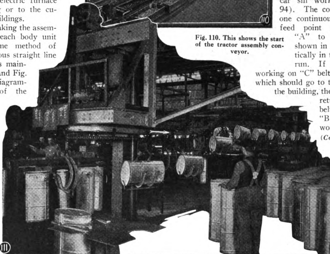
Fig. 111. This is a close-up view showing one of the many I-beam trolley chain conveyors, carrying gasoline tanks from second floor to the tractor assembly lines on first floor.
