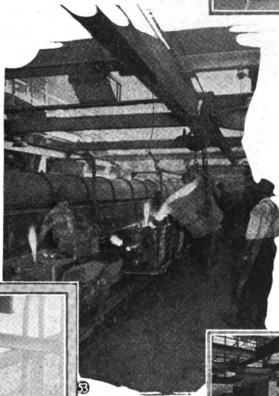
Fig. 52. Enlarged drawing, showing one of the six molding and casting conveyor units, which are an important part of the production equipment of this foundry.
