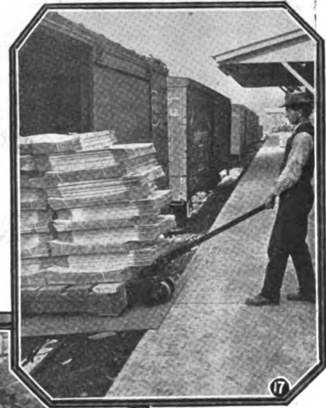
Fig. 17. By using the lift platform system, car unloading costs are materially reduced, as there is no time wasted waiting for truckers.
