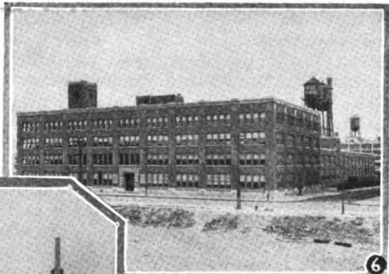
Fig. 6. An unprecedented rush of industries from nearby Manhattan and Brooklyn in the City of New York to Long Island City is caused by its combination of nearness to city population and its open spaces and rail and water facilities. This is the White Truck plant.
