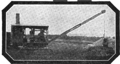
DRAGLINE DREDGES, DIGS, BACKFILLS AND EXCAVATES.
