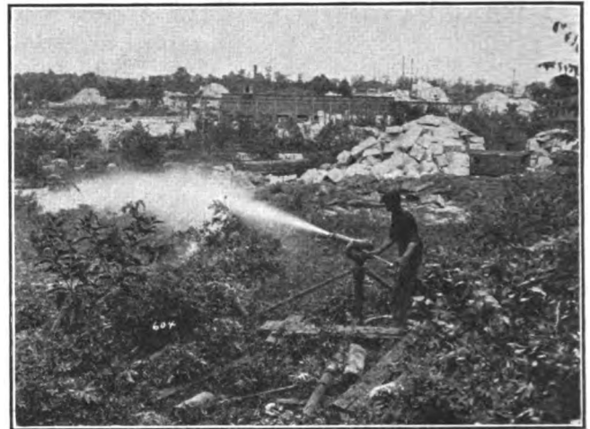
High-pressure stream used to remove the top surface for quarrying.
