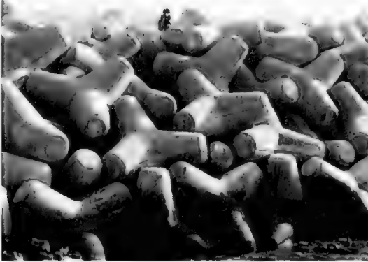
In the Maldives, a reef flat adjacent to the capital of Male was filled using coral rubble and causing sedimentation of nearby reefs. Their degradation was partly responsible for reduced shore protection and extensive flooding in 1987, which resulted in 20-30 per cent of the new infill being lost. Subsequently, artificial breakwaters of concrete tetrapods were installed at a cost of US$10 000 per metre (or US$10 million per kilometre) (Brown, 1997). Not only was this expensive, but it did not prevent serious flooding during the tsunami.
