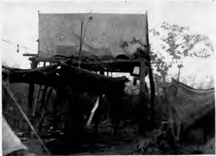
"FIVE SIKH CARPENTERS HAD MADE A STAGING."
