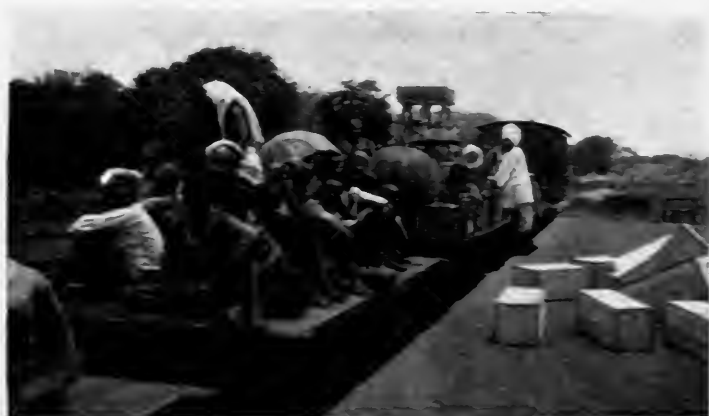
"SEVERAL OF THE TRUCKS WERE HURLED FROM THE RAILS."
