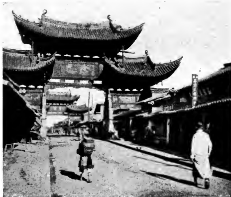
THE EAST-GATE OF YUNNAN FOU.
