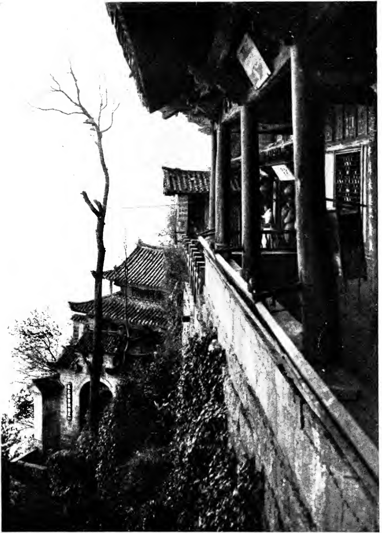
CHINESE ARCHITECTURE ON A STEEP MOUNTAIN SIDE.
