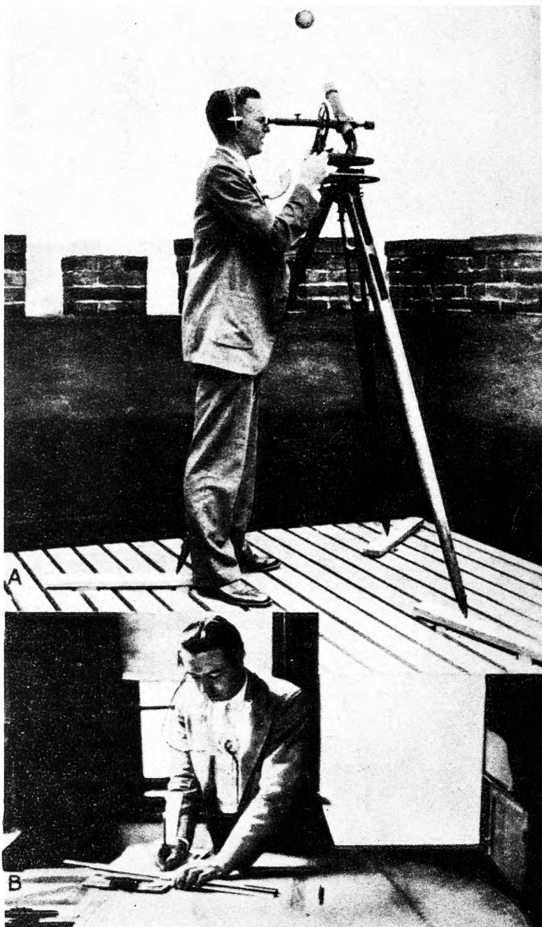
Pilot balloon observation. A, observer following balloon; B, computer at plotting board.
