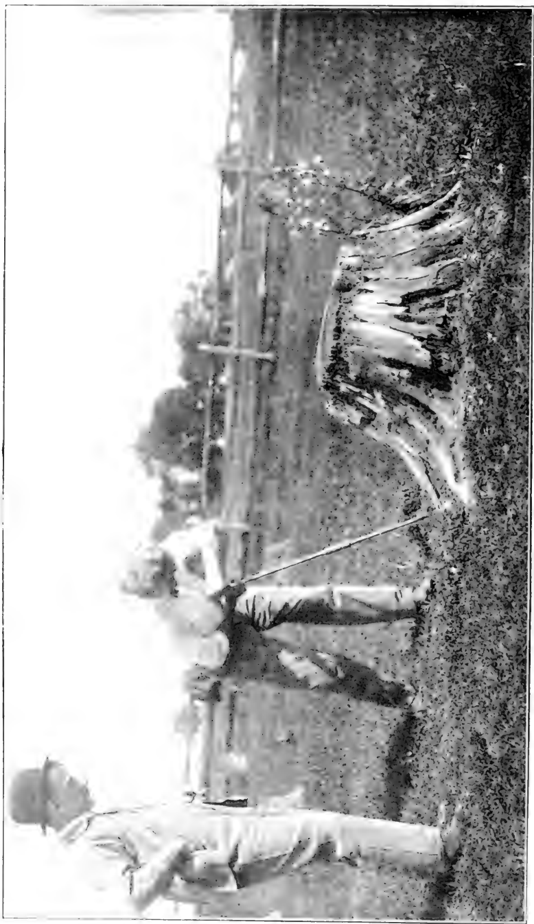
BORING THE HOLE UNDER THE STUMP
