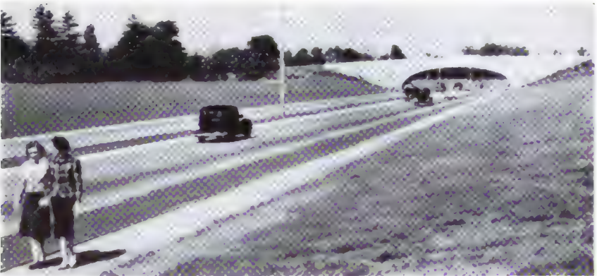
All rural sections of the system carrying traffic of 10,000 or more vehicles daily are located within zones of traffic influence of cities. The above view of Northern State Parkway at Westbury, Long Island, is fairly representative of the type of construction proposed. Costs may range from $150,000 to $700,000 per mile, depending largely upon right-of-way expense.
