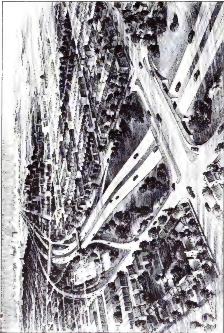
PLATE X.—Built within a block-wide right-of-way, on a gently rolling grade, depressed to pass under bridges at important cross streets and rising to normal ground level between, with varied median strip width and use of border areas for suitable neighborhood recreational purposes, a section of the interregional system traversing residential areas of a city, conforming in all respects to standards proposed by the committee, is shown in this sketch.
