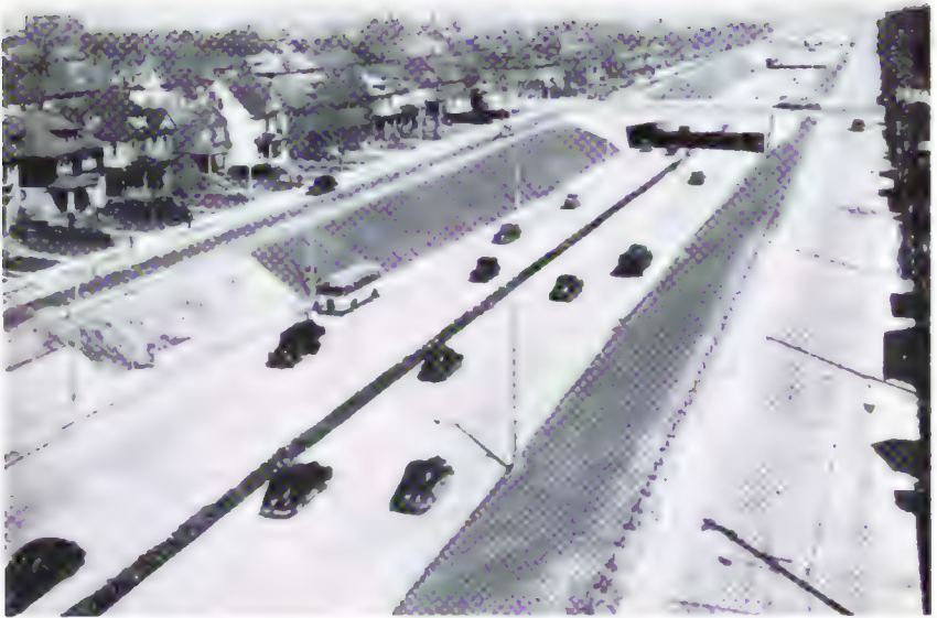
A former street has here been preserved to form the local service way at the left. The right service way abutting the rear of properties facing on the next street is built on part of a half-block strip acquired for the improvement. The right-of-way is inadequate for the type of development proposed by the committee.
