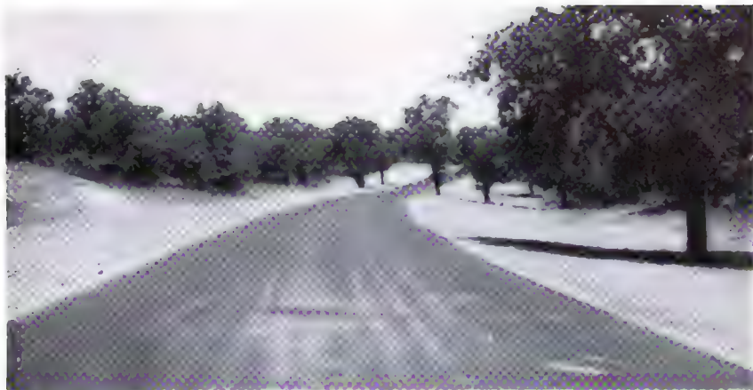
For sections of the system designed for traffic of less than 1,000 vehicles per day, this picture of an existing road in Texas typifies the character of construction proposed. Consisting of a single 24 foot pavement of appropriate material, with wide shoulders and easy slopes, such sections can probably be constructed at costs ranging between 40 and 60 thousand dollars per mile, depending mainly upon the quantity of grading and the number of grade-separated intersections.
