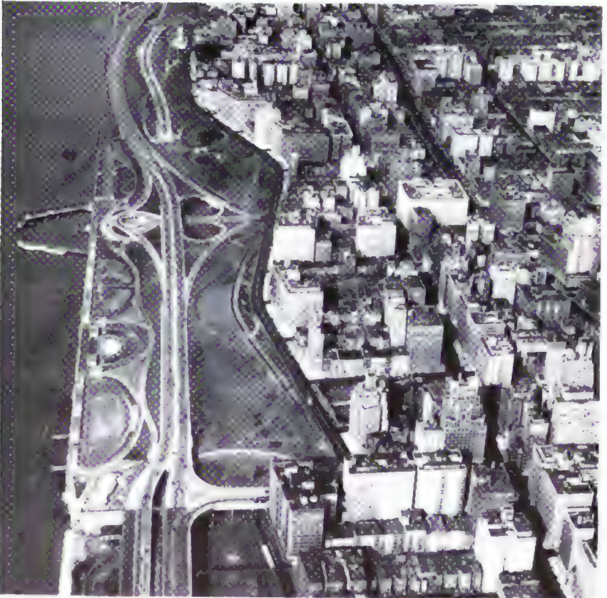
PLATE I.—An urban express highway constructed over railway tracks. The upper view shows construction in progress on the highway deck over New York Central Railway tracks. The lower view shows the completed and landscaped Henry Hudson Parkway built over the tracks.
