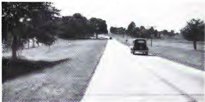
Sections of the system designed for traffic of volumes between 1,000 and 2,000 vehicles per day should be similar in most respects to those serving smaller traffic volumes, but surfaced with pavements of higher type. Cost may range between 50 and 70 thousand dollars with variations in grading quantities and number of grade-separated intersections. The Alabama highway pictured above conforms approximately to the standards proposed.
