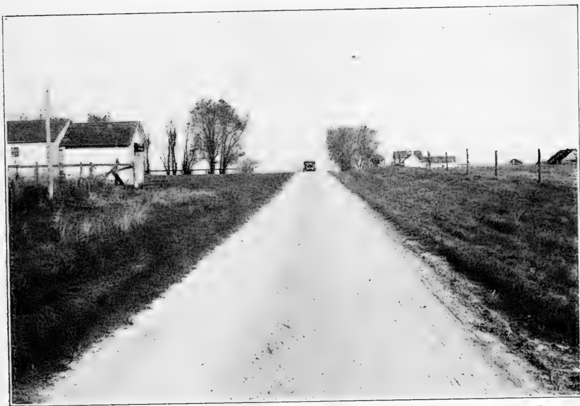
A GOOD ROAD. Typical of the best gravel road in Greene County, Iowa, which has been in use for seventeen years with no new gravel and no work upon it except road dragging in the spring. No mud has ever come through it. Graveling road of this width in this County averages $350 per mile.— Iowa State Department of Education.
