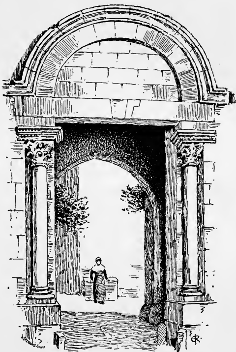
SOUTH ENTRANCE TO THE CLOISTER, ARLES CATHEDRAL.
