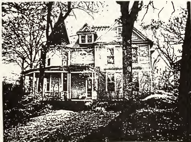
Fig. 8 The Markham House on Cleveland Street. Demolished, 1972. Reprinted from A Pictorial History of Durham , Joel and Frank Kostyu.
