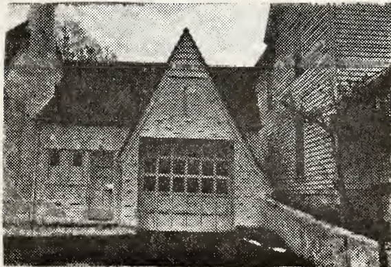
138. Mill Park Gas Station. 1200 East Main Street. 1929 Whimsical early gas station addresses all streets from corner site. Three sided, painted, skinteled brick one-story building. Steeply gabled blue ceramic tile roof; two exterior end chimneys. Picturesque French chateau image, typical of Pure Oil stations of twenties and thirties. Three parts of building include two garage wings with tin ceilings and angled central office.
