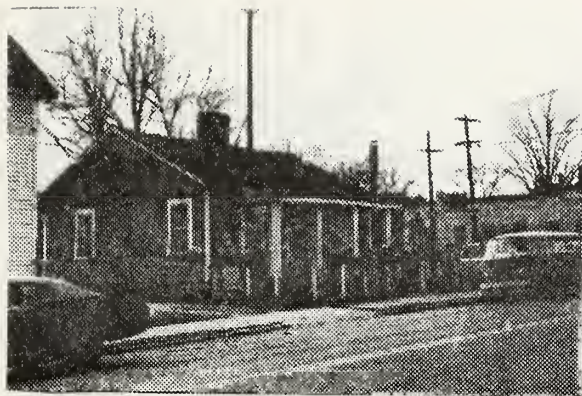
150. 209 South Holman Street and 1302 Angier Avenue. 1913-1937
