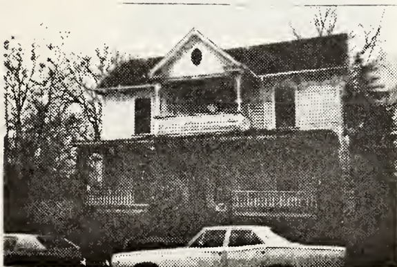
95. 1102 Angier Avenue. Pre-1913 This large "I" house has a front porch with a covered second story pedimented balcony, Italianate trim, and originally had 2 exterior rear chimneys and a 2-story "ell" wing, 2/2 sash and replacement doors. Was a single family and now multi-family. Good shape and worth saving.
