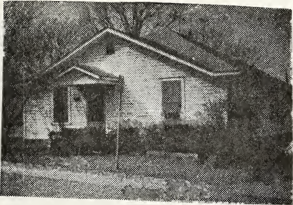
136. 115 North Holman Street. 1913-1937 One-story house with hip roof, front cross gable, central chimney, German siding, 9/1 sash windows, and replacement front door. Apparently front porch was later enclosed and a modern stoop added.
