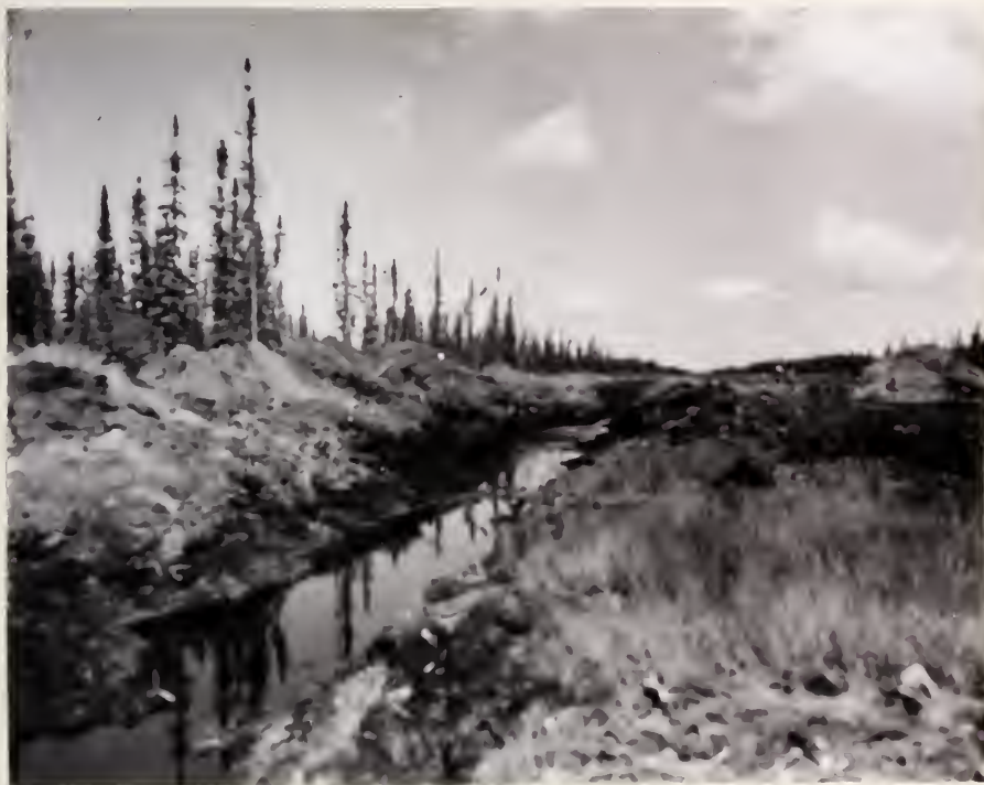
Fig 1 - Ditch blasted in Muskeg near Mile 253 Alaska Highway
