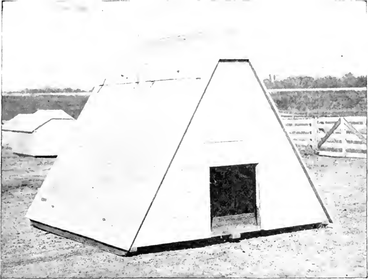
Fig. 22. "A" House (Doors Hinged at Top). Front view showing improved ventilator: closed. Top eye bolts should be nearer ridge. Make the doorway higher for mature swine.
