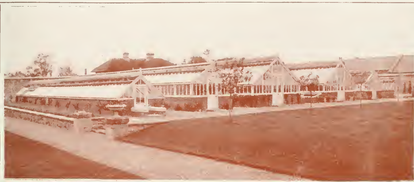
ERECTED FOR THE RT. HON. THE EARL OF DUNRAVEN, ADARE MANOR, CO. LIMERICK
