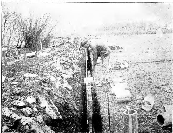
Fig. 162. Placing tile with tile hook.
