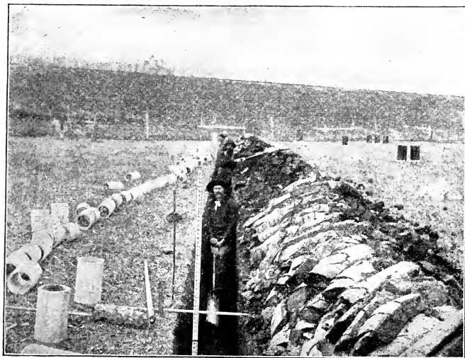
Fig. 160. Removing the last two spadings from the ditch.
