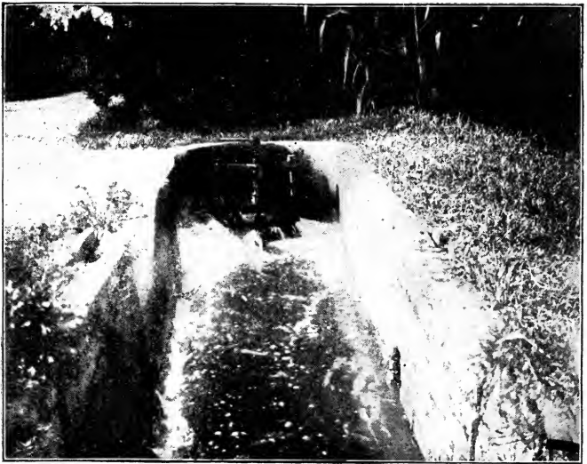
Fig. 127. Sewage hydrant at Gennevilliers.
