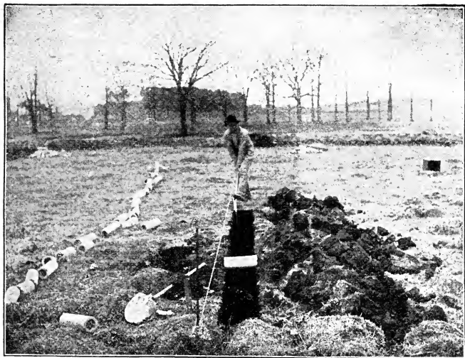
Fig. 159. Commencing a ditch.
