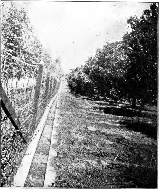
Fig. 107. Head ditch or cement flume for orange orchard, Redlands, California.
