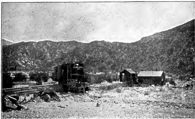
Fig. 66. Submerged dam at San Fernando, California.
