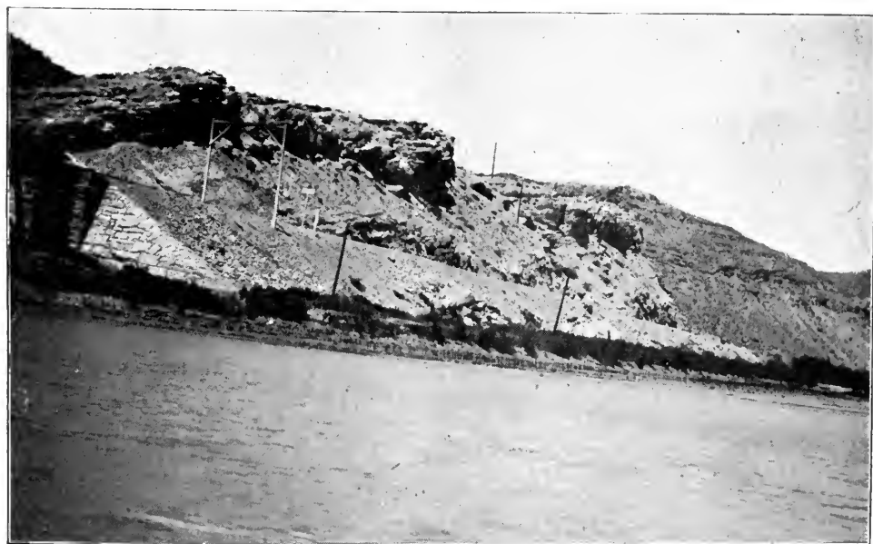
VIEW OF MEXICAN SIDE SHOWING RAILROAD TRACKS THAT WILL BE REMOVED.
