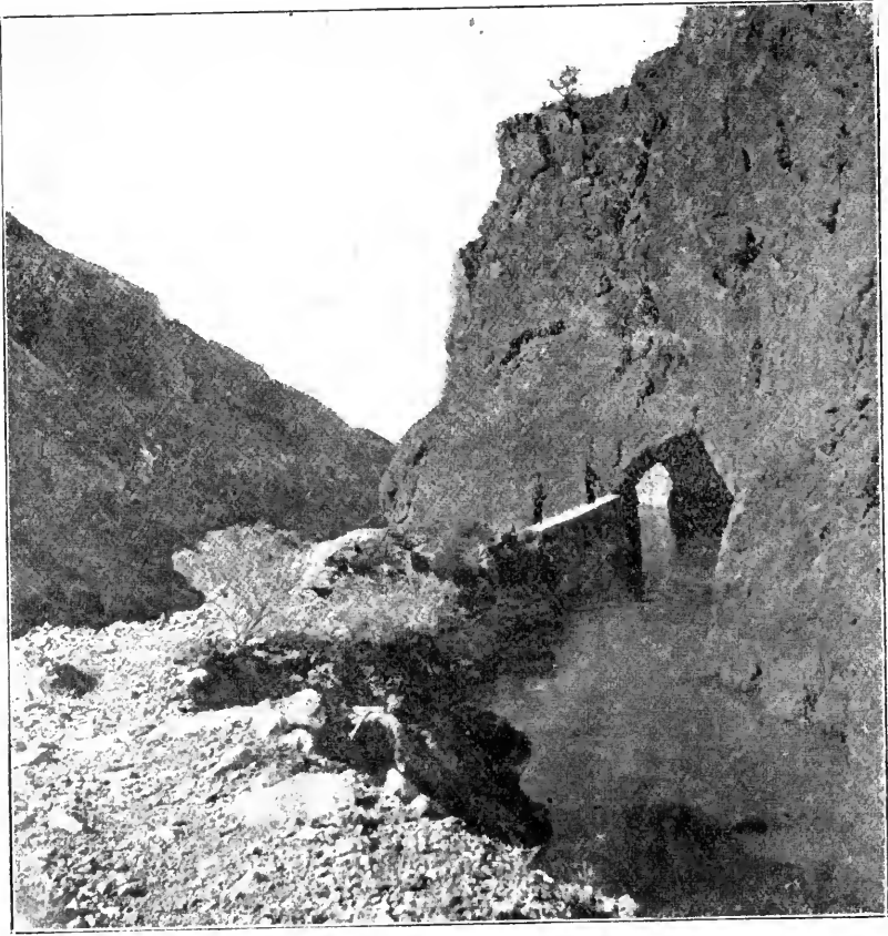
BEAR RIVER CANAL, SHOWING STONE CUT AND TUNNEL.
