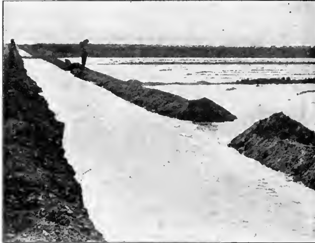
FLOODING THE LAND AT IMPERIAL.
