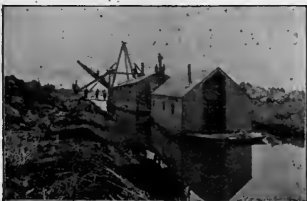
One-yard Ditching Dredge.
