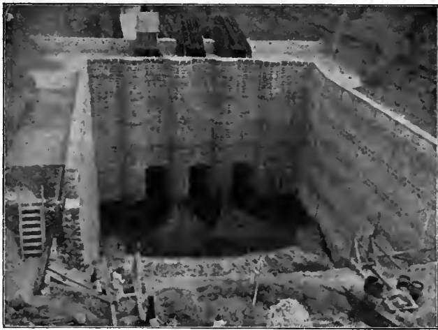
REAR ELEVATION OF DAM.
