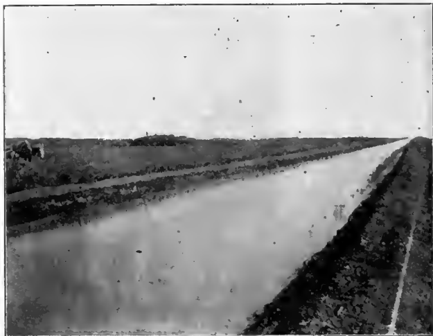
VIEW OF MAIN CANAL, IMPERIAL.
