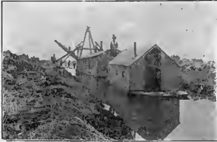
One-yard Ditching Dredge.
