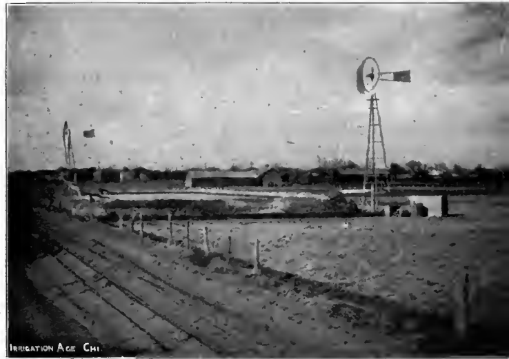
IRRIGATION MILL AND RESERVOIR.
