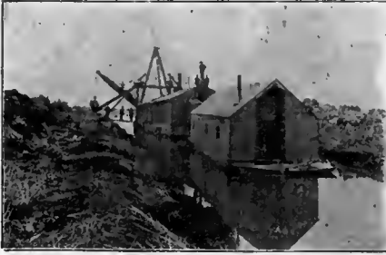
One-yard Ditching Dredge.
