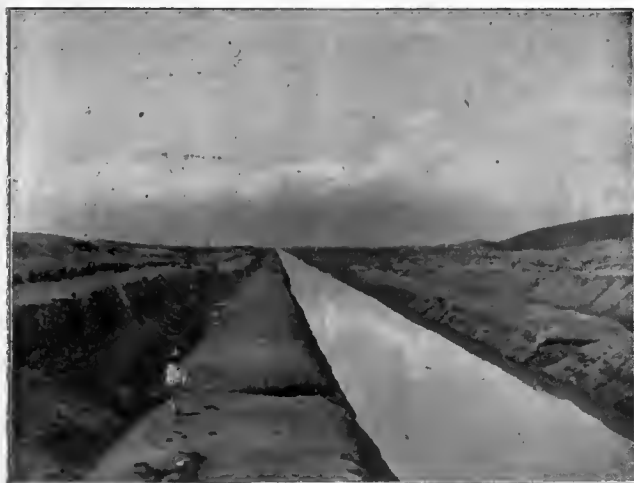
MAIN CANAL UP STREAM. 22ND MILE.
