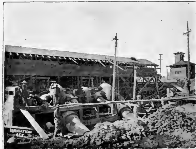
PARTLY COMPLETED BUILDING. PUMPS IN FOREGROUND.
