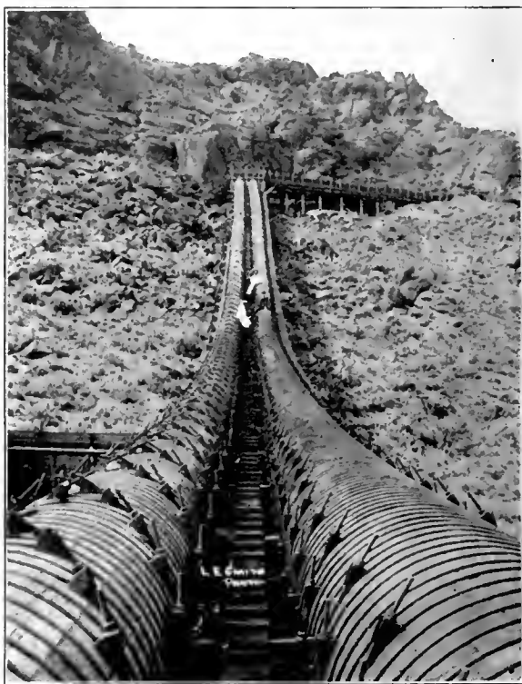
Inverted Syphon, Condon Irrigating Ditch, three miles from North Yakima, Wash., on Northern Pacific Railway.
