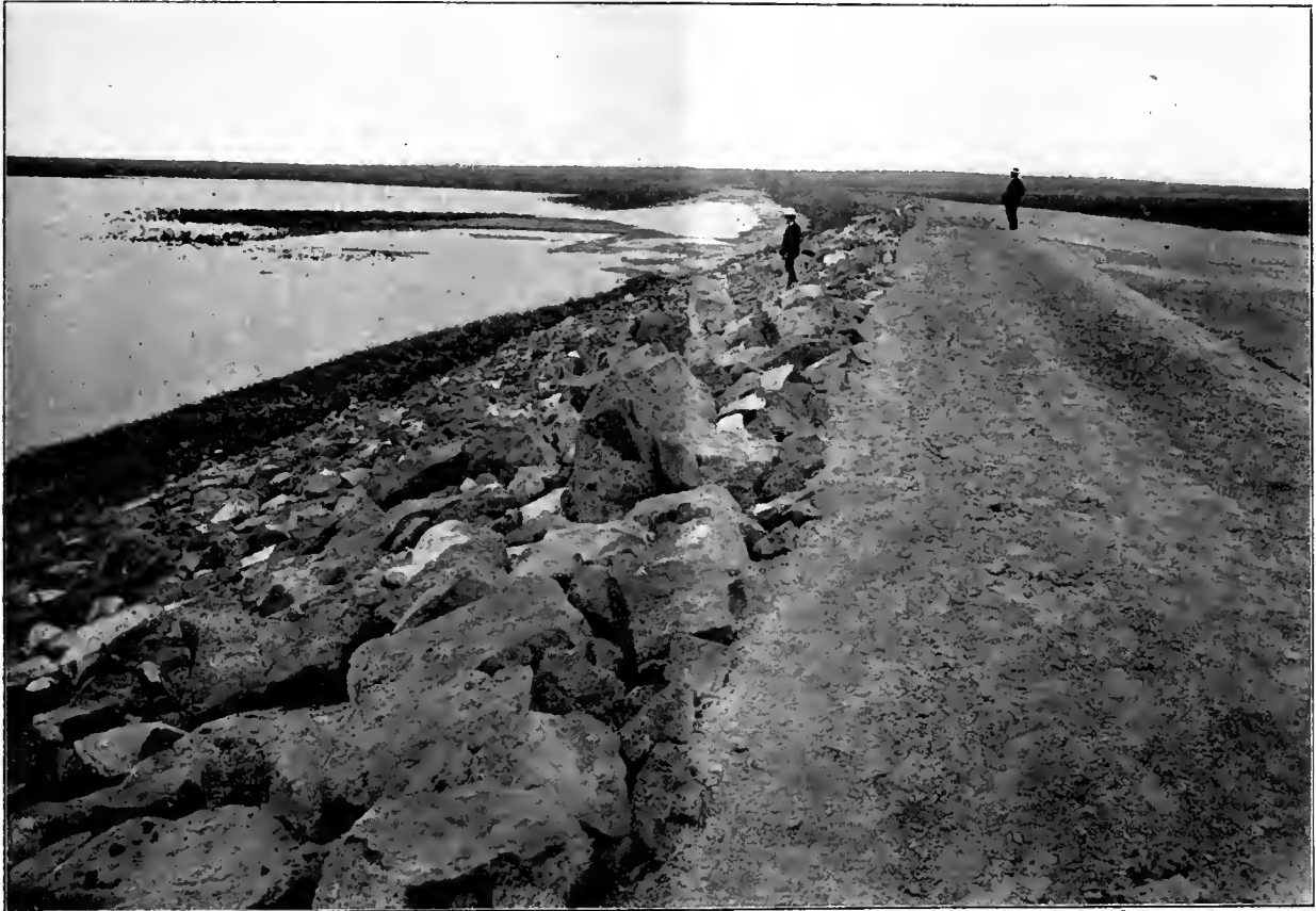
Dry Creek Reservoir, Twin Falls Land & Water Co., Lincoln County, Idaho.
