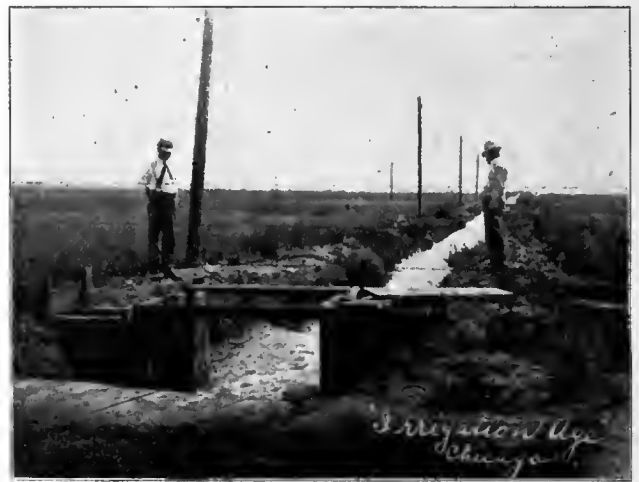
One of Laterals from Canal of Billings Land and Irrigation Co. East of Billings.
