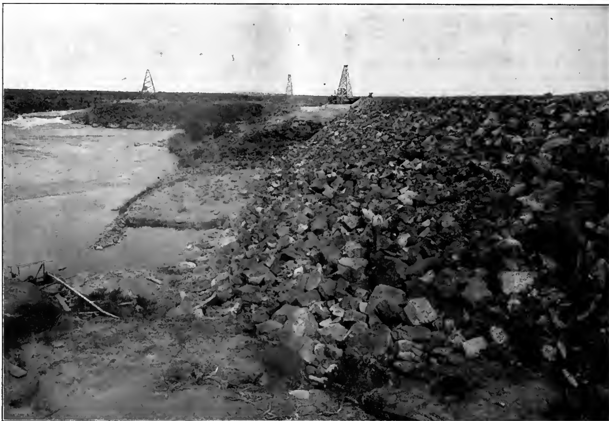
Diversion Dam at Milner, Idaho, Twin Falls Canal.
