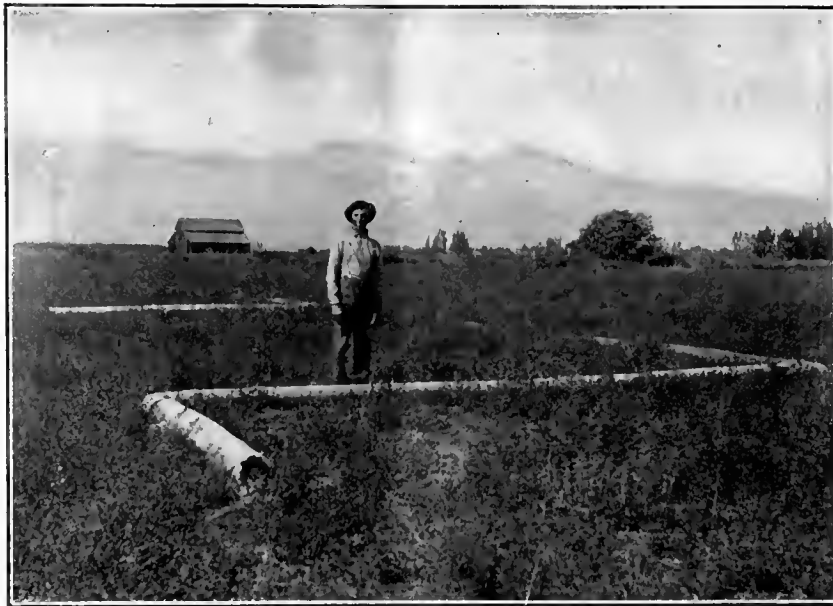
Distributing Water From Sections of Metal Pipe Attached to Main Pipe by Canvas Elbows.
