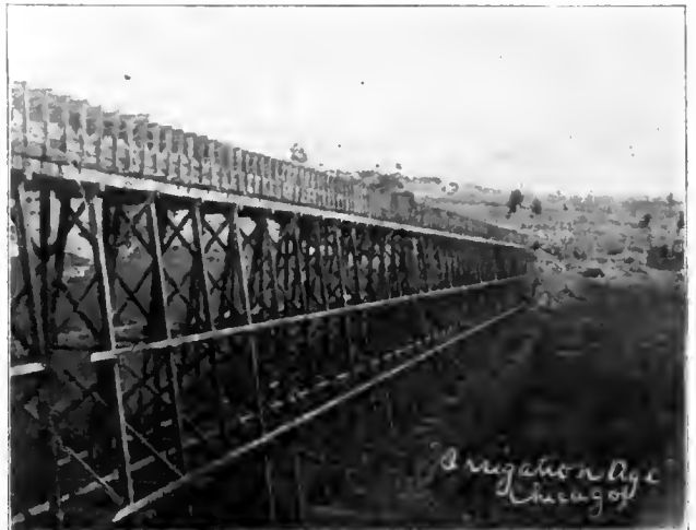
Trestle carrying Flume of Billings Land and Irrigation Co.'s Canal. This Flume receives water soon after it leaves tunnel shown elsewhere in these columns.
