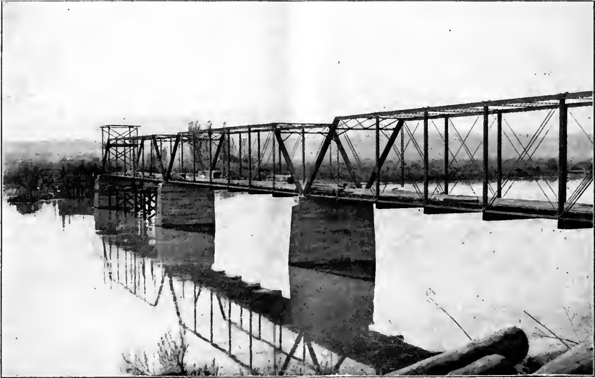
Weiser Bridge, across Snake River, Weiser, Washington County, Idaho.
