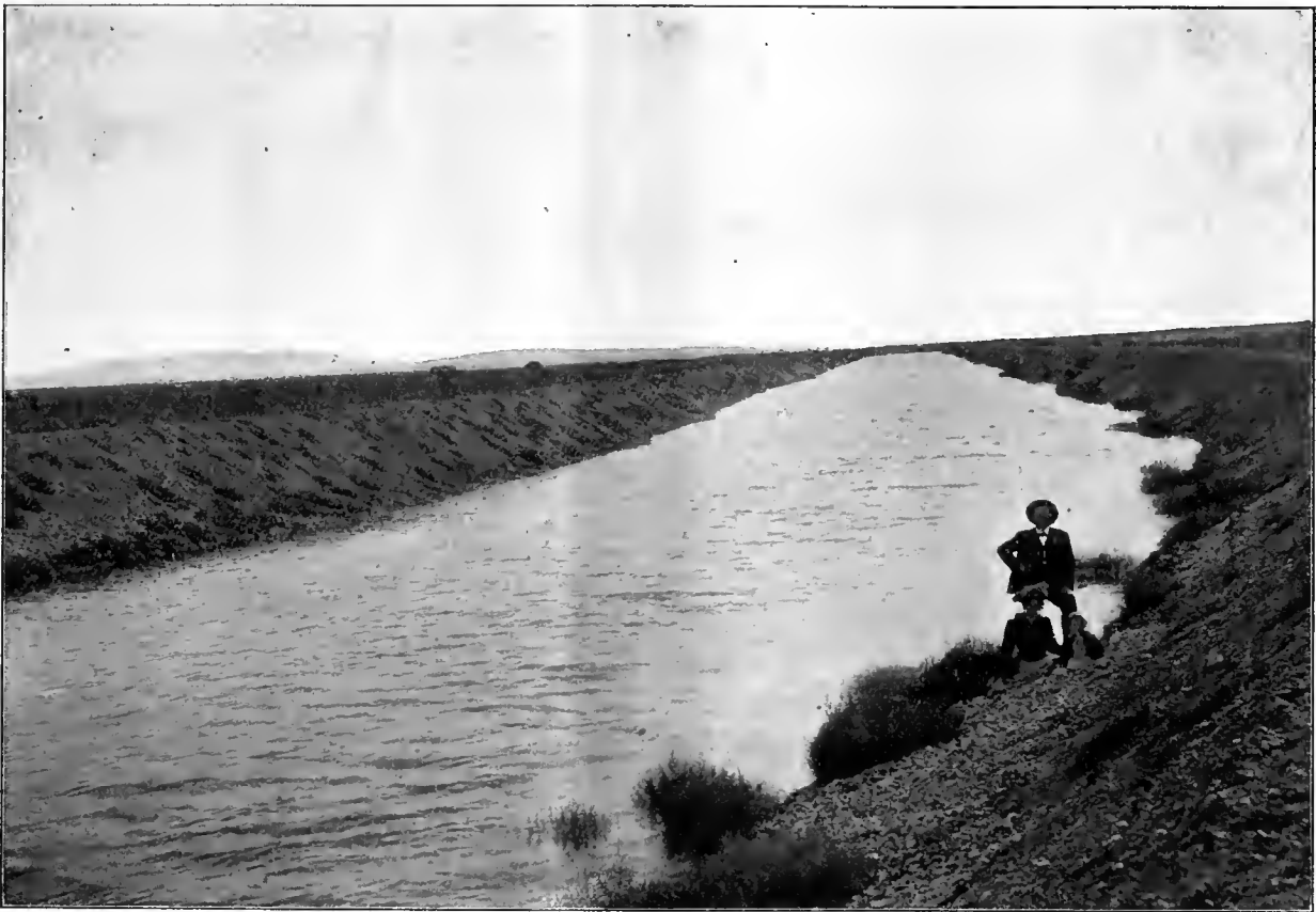
American Falls Irrigation and Power Company's Ditch, near Morehead, Bingham County, Idaho.
