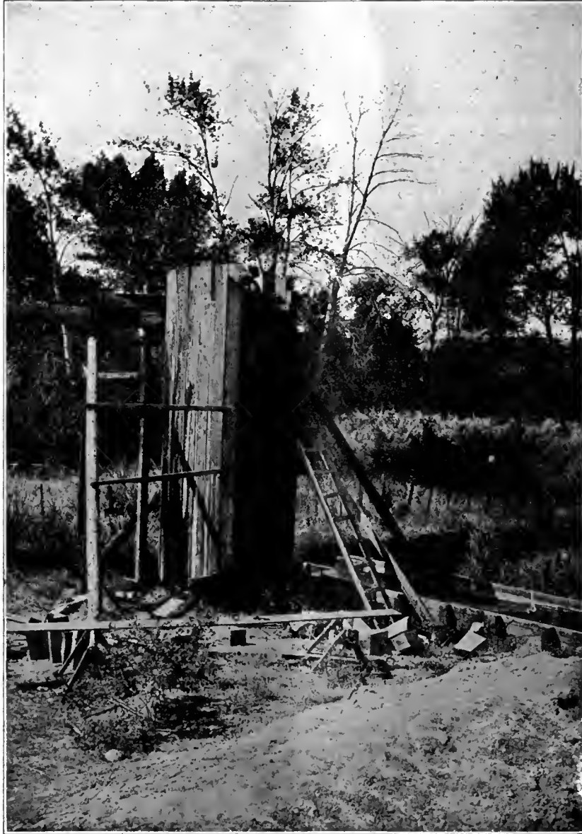
Chain and Bucket Operated by Overshot Wheel, Selah, Washington.
