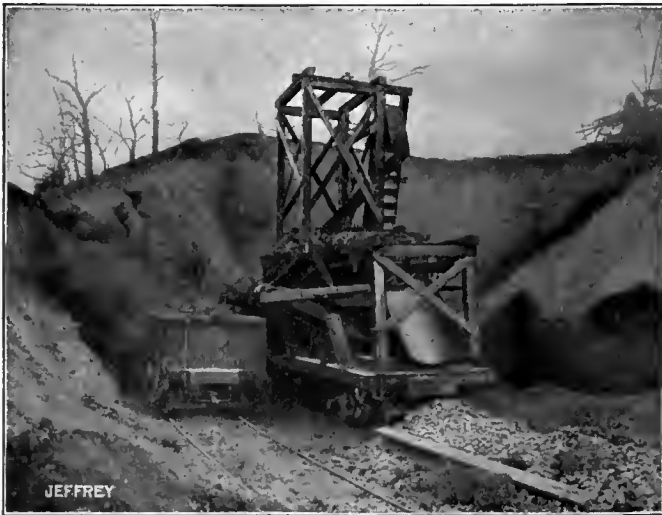
Elevator and Screening Machine for handling Gravel.
