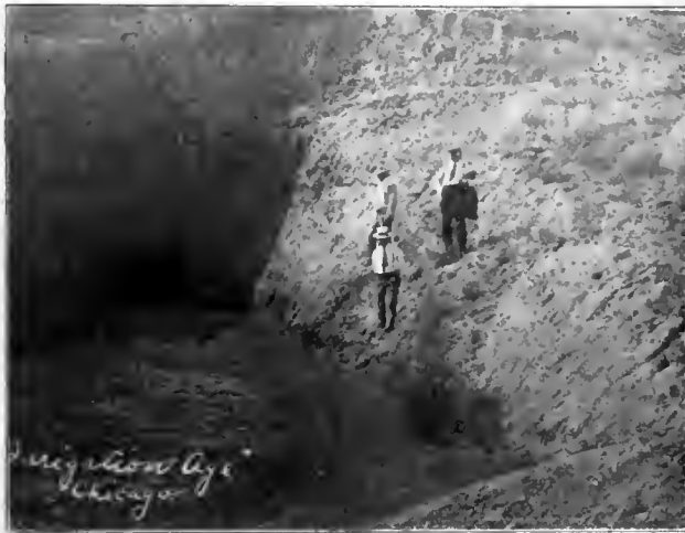
Mouth of 1,800-foot Tunnel carrying water through rock cliff near Billings.
