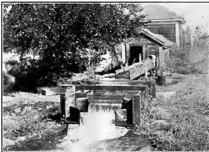
A MEASURING WEIR.
