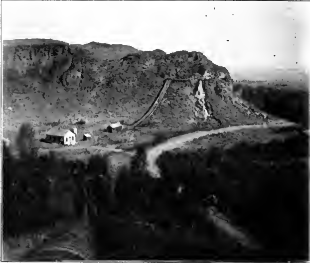
Great Irrigation Syphon one-half mile in length. The water falls 100 feet from the mountain side in distance and runs up the mountain side in immediate foreground emptying into the flume shown in another illustration. Near North Yakima, Wash., on Northern Pacific Railway.
