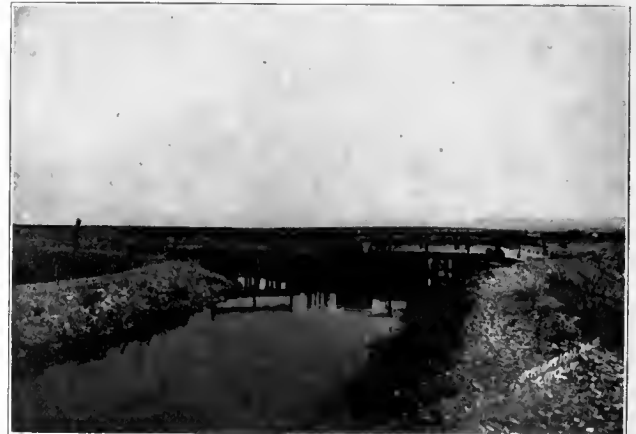
Northern Pacific Irrigation Canal, Kennewick, Wash., Dividing Gates Main Canal on right, Lateral No. 2 on left.
