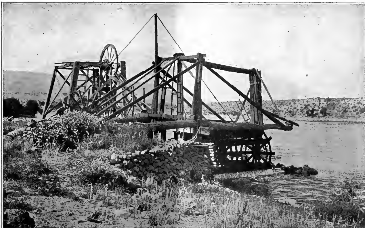
Wheel Operating a Rotary Pump, Yakima River, Washington.
