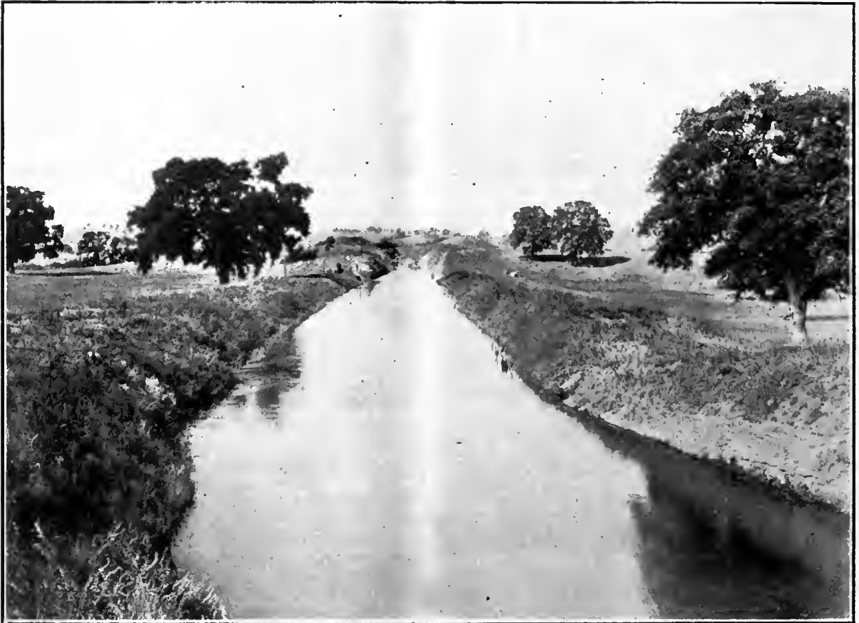
A CALIFORNIA IRRIGATION CANAL IN THE FOOTHILLS With a high duty of water running in the canal should irrigate 50,000 acres.
