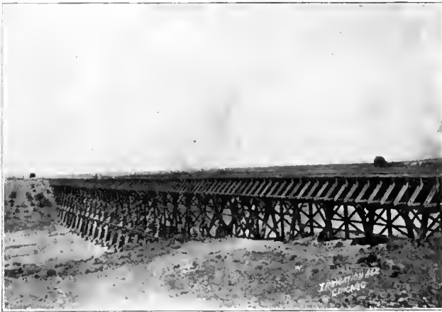
Trestle at Badger Canyon Flume No. 2 Northern Pacific Irrigation Canal, Kennewick, Wash.
