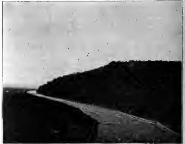
The Flume into which the great syphon empties and runs around the mountain 85 feet above the country road.
