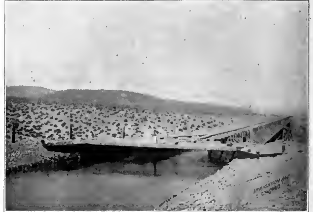
Bridge and Flume Northern Pacific Irrigation Canal, Kennewick, Wash.
