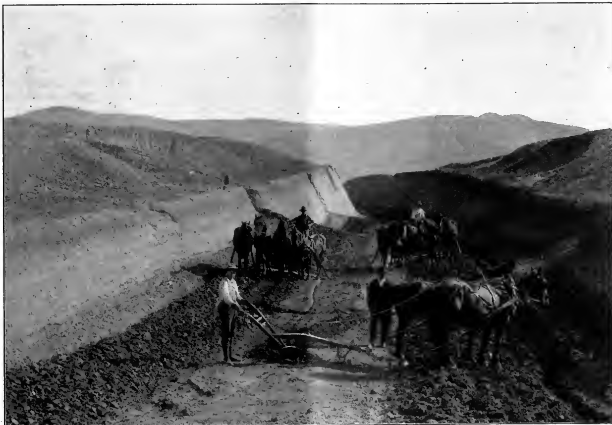
Big Cut, on Mink Creek Canal, Oneida Irrigation District, Idaho.
