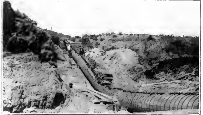
Showing Construction of Pipe Line.
