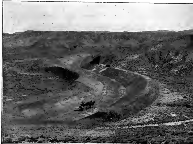
Completed Section of the South Side Canal, Uncompaghe Valley, Colo.
