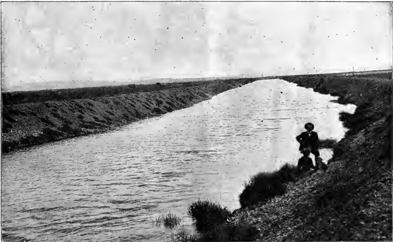
SECTION OF MAIN CANAL, SIXTEEN MILES FROM HEADGATE
