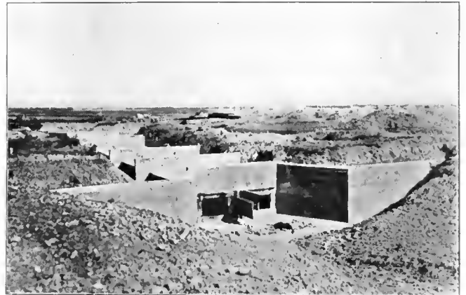
Concrete culvert on main canal.
