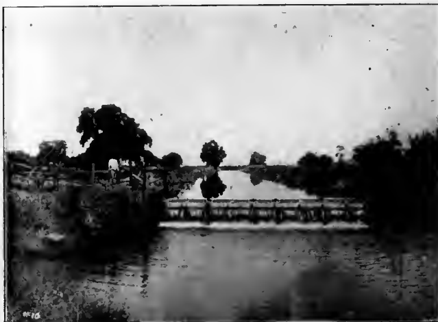
Weir in main canal, Butte county, California.
