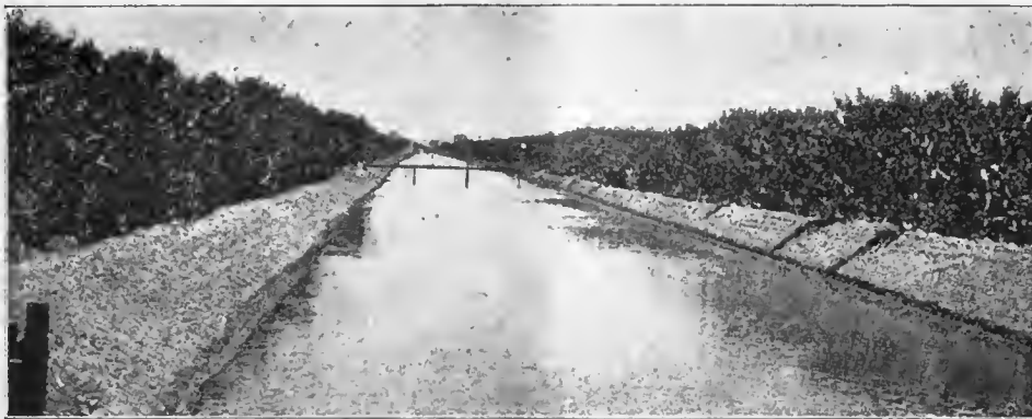
Main Canal supplying water to Gridley and Sunset Colonies
