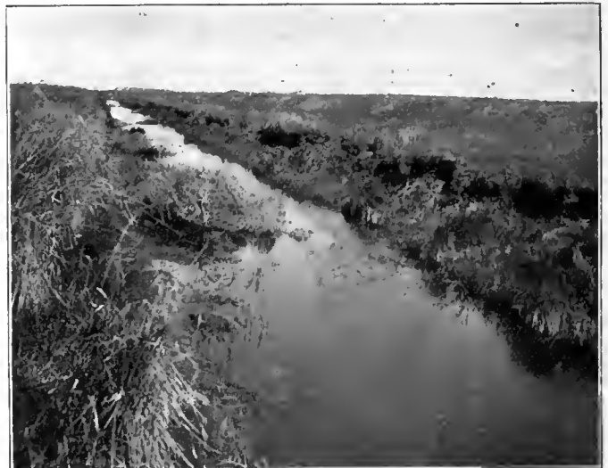
An illustration of a three-year-old ditch built by dipper dredge in northwestern Iowa, showing banks caved practically throughout their entire length and demonstrating why ditches built in this manner require frequent reconstruction.
