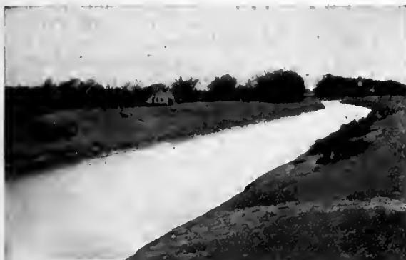
Irrigation Canal near Garden City, Kas.
