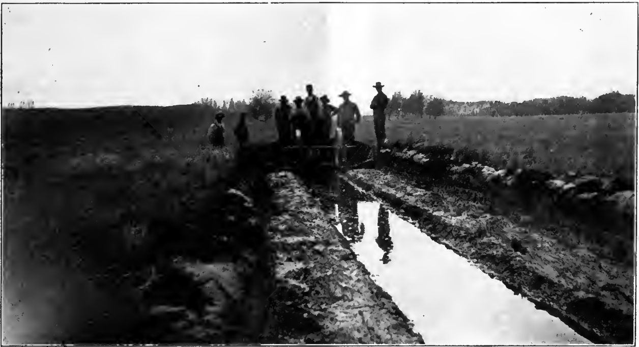
Edward's Ditching Machine in Operation.
