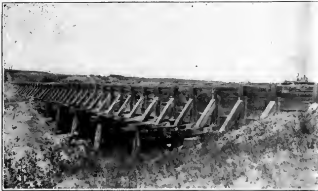
One of the Flumes on Main Canal.
