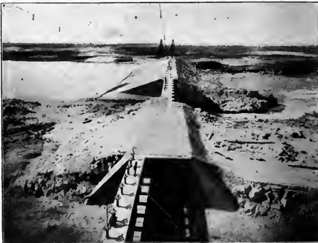
Minidoka Dam and Regulating Devices. View from north end. August 29, 1906. Minidoka Project, Idaho. Photo by F. C. Horn.
