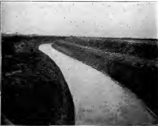
Photograph of a ditch one year old constructed by the Austin Drainage Excavator, demonstrating that ditches constructed in this manner maintain their original shape and become permanent waterways.
