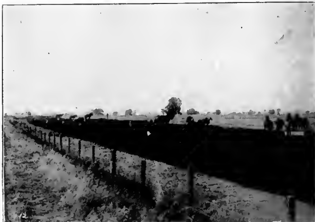
Building Main Canal, Sutter county, California.
