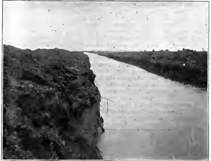
A recently constructed ditch built with dipper dredge, showing the vertical banks and waste banks constructed immediately adjacent to the ditch and demonstrates why ditches constructed in this manner cave and are filled by erosion in a short time.
