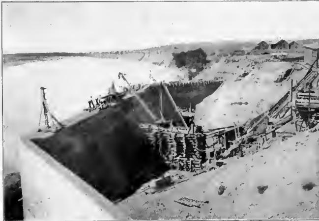
Headgates structure, nearly completed.
