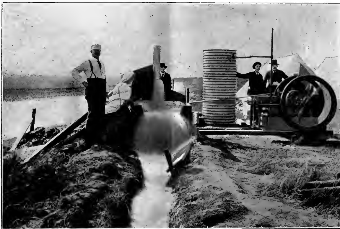
This cut shows a 10 horse power gasoline engine pumping water for irrigation near Garden City, Kansas. This engine was manufactured and installed by the International Harvester Company of America, whose headquarters are Chicago.
