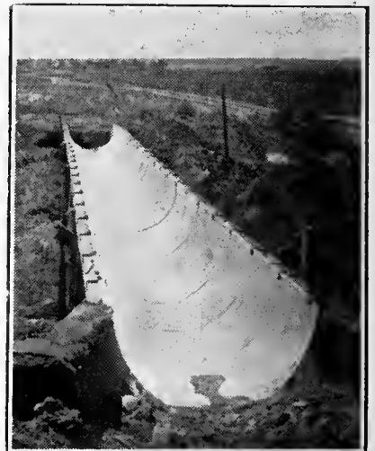
Leavitt Flume on North Extension Ditch near Greeley
