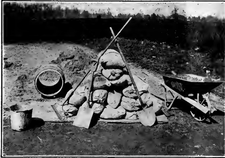
Cement on the Work Piled Properly on Wooden Platform.
