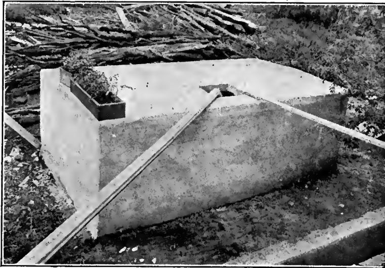
A Farm Cistern Built on a Three-Foot Terrace.
