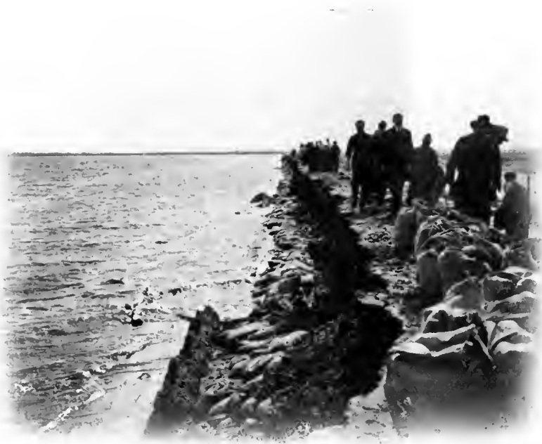
Fig. 7. Lower Latham Reservoir, Greeley, Colo. Destruction by Wave Action, April, 1912.
