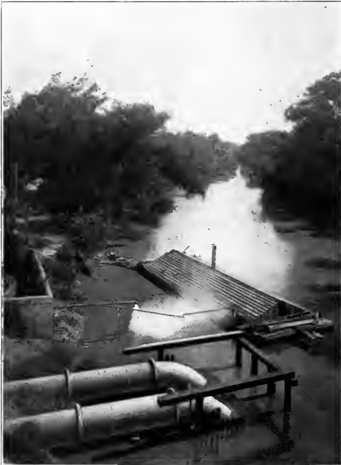
Fig. 2. Oil Barge Unloading. Suction Pipes for One of the Pumps and Protective Cribbing. View of Stream Supplying Water for the Pumps.
