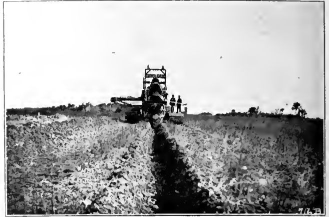
Cutting Ditch in Imperial Valley.
