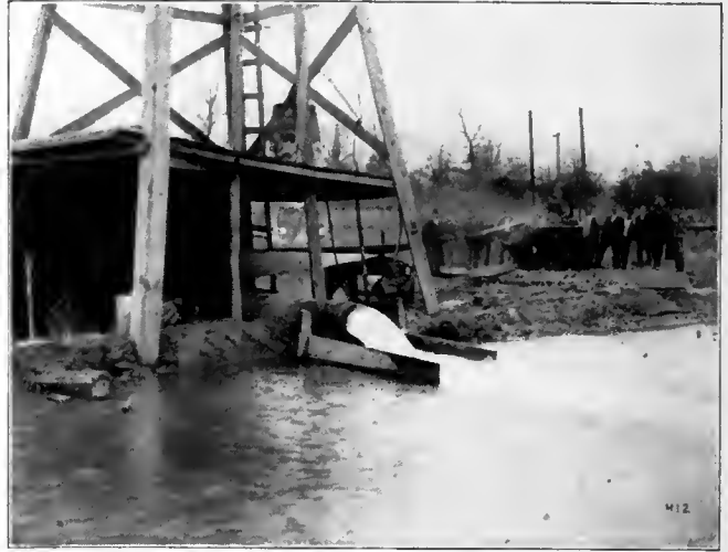
Oil Pull "E" Motor Pumping 2,000 Gallons Per Minute.
