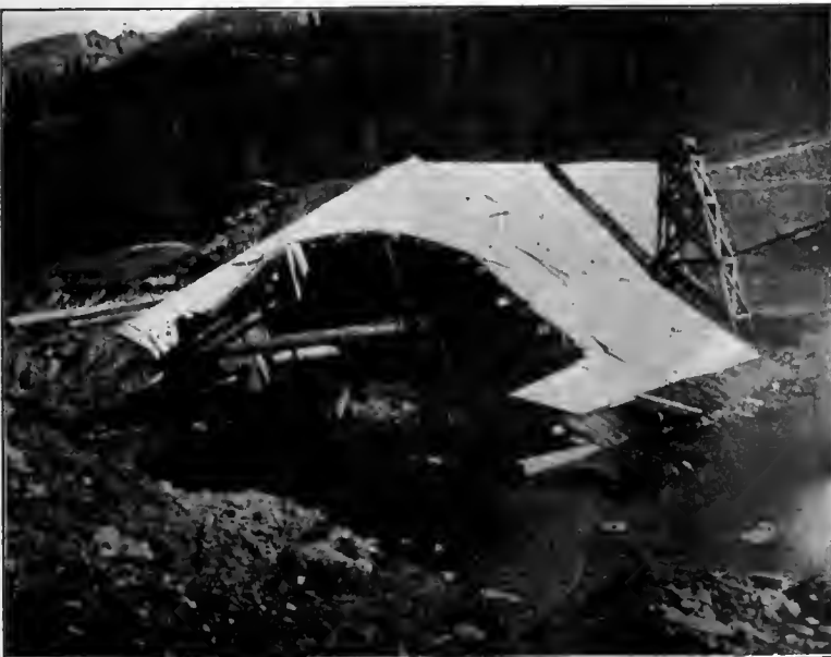
Fig. 10. Telluride Power Co. Break, October 2, 1909.
