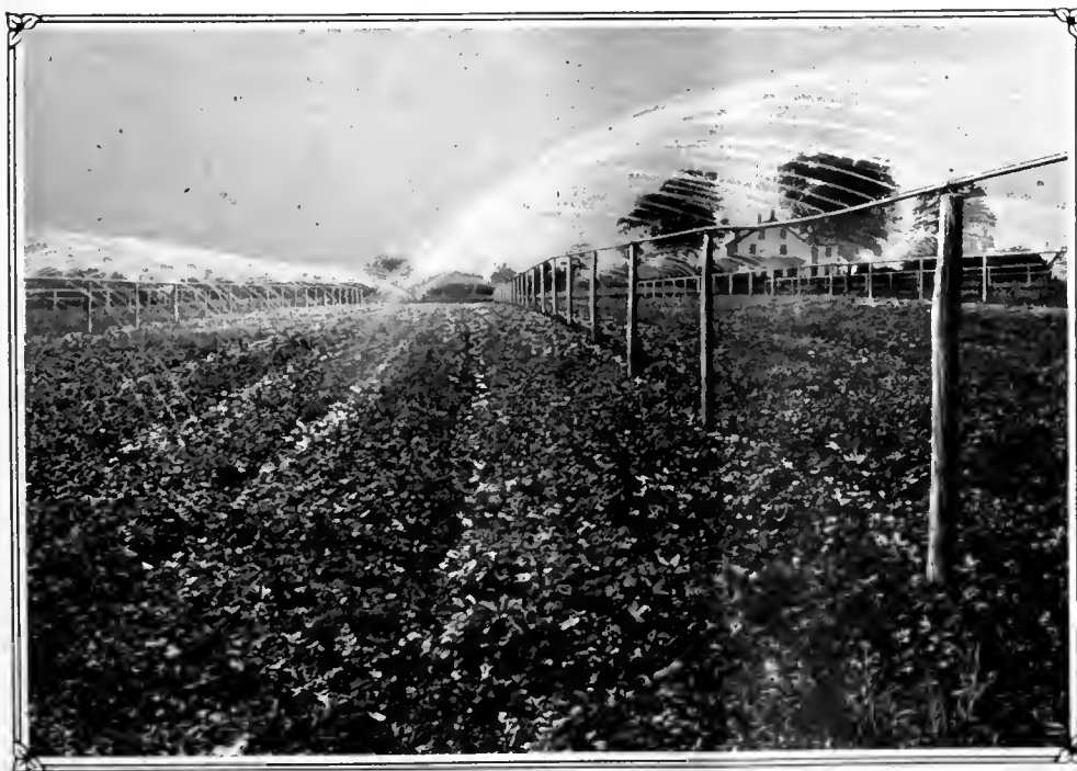
Irrigating a Strawberry Patch. This System Extends Over Five Acres at Rancocas, N. J. Nozzles Every Four Feet on Lines Fifty Feet Apart. The System Distributes 250 Gallons of Water a Minute.
