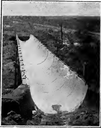
Leavitt Flume on North Extension Ditch near Greeley
