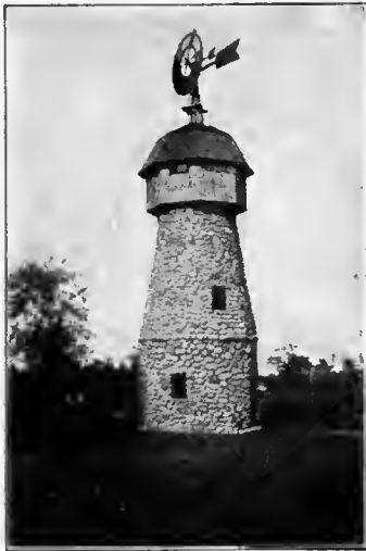
The Eclipse is always artistic. Many farm homes utilize the windmill to secure a water pressure system. The above shows an especially attractive installation of this kind.
