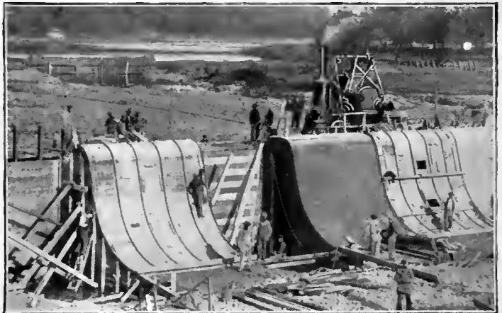
Front view, showing section of finished dam at Milan, Ill.
