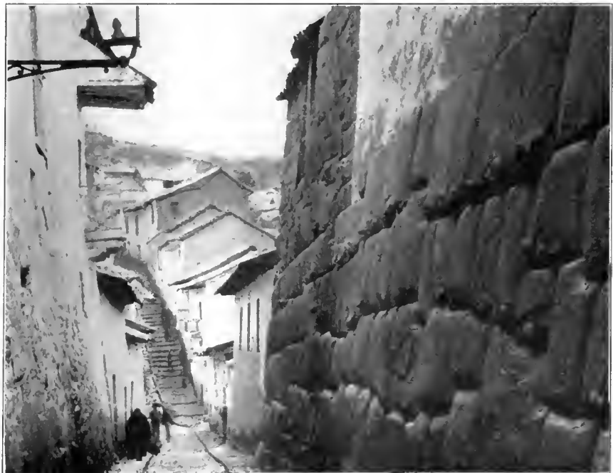
Street in Cuzco Showing Old Inca Foundation.
