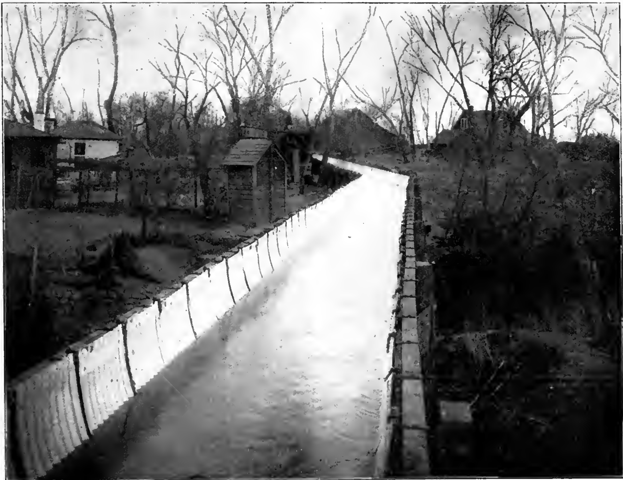
A No. 98 Flume Erected for the Stratton Estate, Colorado Springs. Capacity 40 Cubic Feet Water per Second on a Grade of Five Feet to the Mile.
