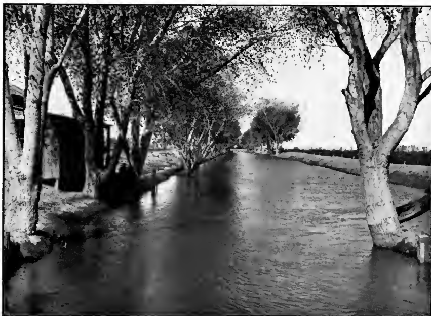
Irrigating Canal, Salt River Project, Arizona.
