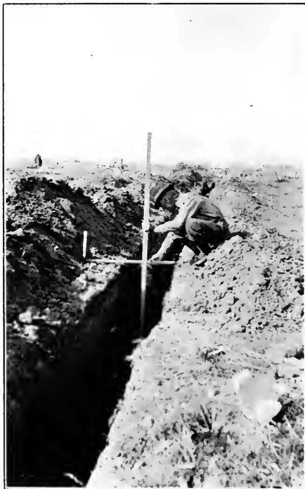
Fig. 3—Drainage system under construction. Note depth of trench.
