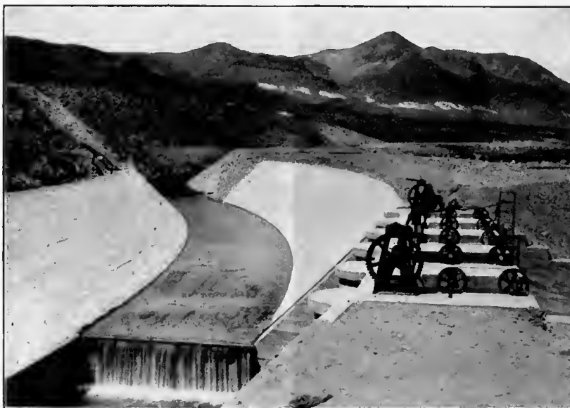
Concrete Lining and Distributing Gates. Canal of Truckee-Carson Project, Nevada.
