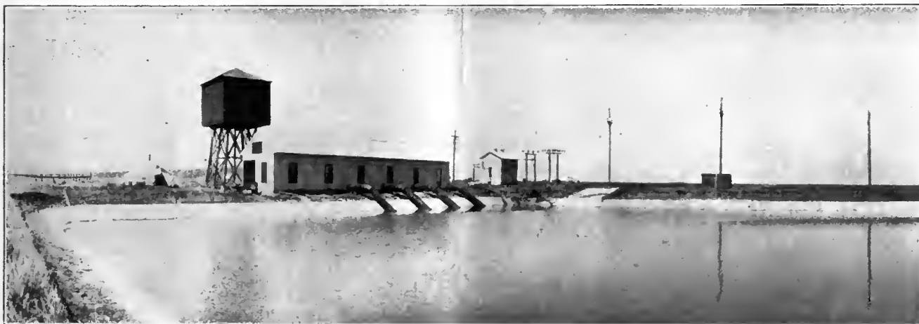
One of the Pump Stations on Patterson Irrigated Farms, Patterson, California. There Are Eight of These of Varying Capacity on This Project.
