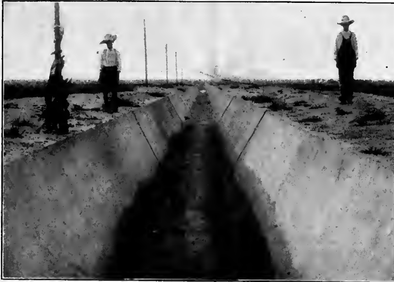
Concrete Lined Canal, Garden City, Kansas, Irrigation Project.
