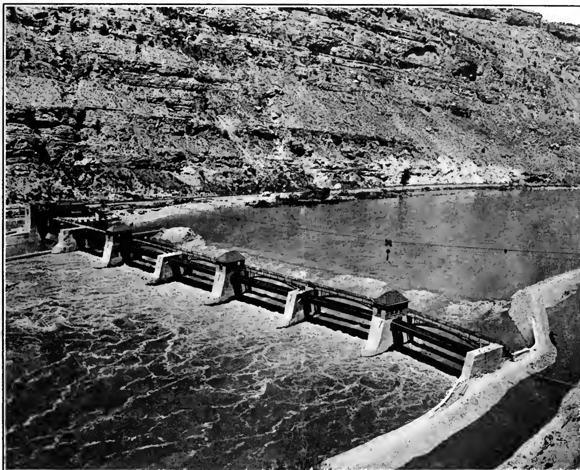
Roller Crest Diversion Dam, Grand Valley Project, Colorado. This dam is constructed on a comparatively new principle and is performing its work satisfactorily. This structure was erected under the supervision of Project Manager and Engineer J. H. Miner and will stand as a monument to the ability of this capable gentleman.
