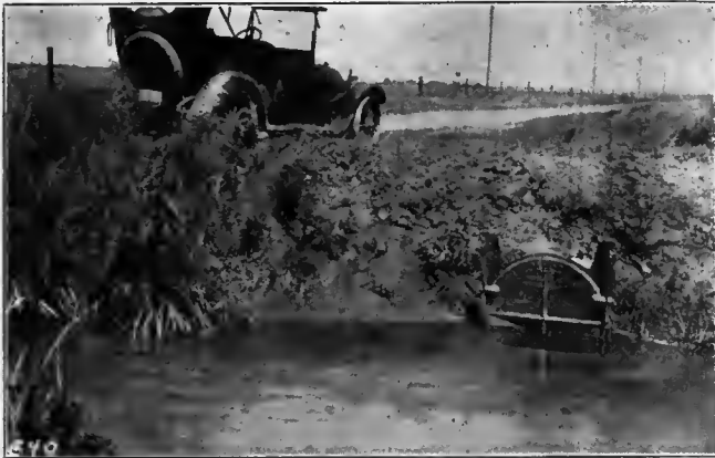
Automatic Drainage Gate Attached to Corrugated "Armco" Iron Pipe.
