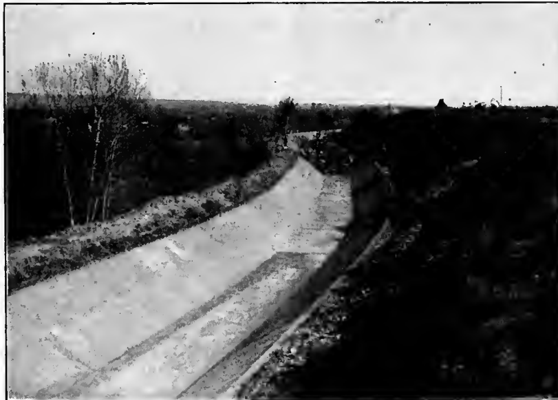
Construction Work in Progress on the Ridenbaugh Canal, Idaho.
