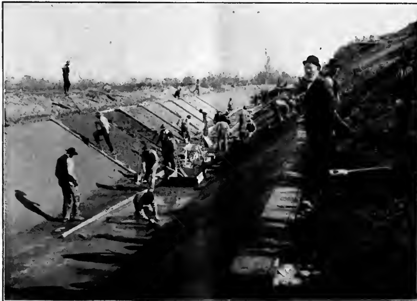
Cement Construction on Irrigation Work.
