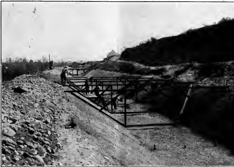
Cement Construction on Irrigation Work.
