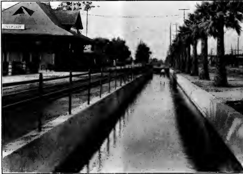
CONCRETE IN IRRIGATION CANAL CONSTRUCTION
