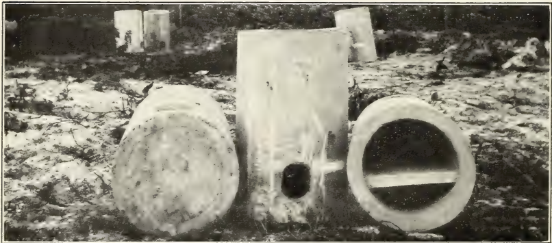
FIG. 2.—SUBIRRIGATION STOP POCKETS, SANFORD, FLA.
