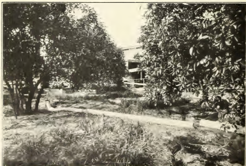
FIG. 2.—SIX-INCH CAST-IRON IRRIGATION VALVE AND HOSE CONNECTION TO SLIP-JOINT PIPE FOR IRRIGATING ORANGE GROVE, PALATKA, FLA.
