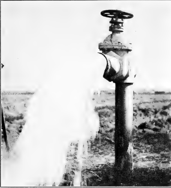
FIG. 1.—FLOWING WELL AT HASTINGS, FLA., USED FOR SUBIRRIGATION.
