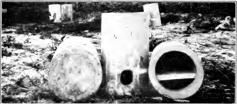
FIG. 2.—SUBIRRIGATION STOP POCKETS, SANFORD, FLA.
