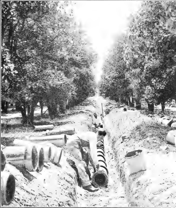
FIG. 1.—LAYING VITRIFIED TERRA-COTTA PIPE IN CITRUS GROVE, ORLANDO, FLA.
