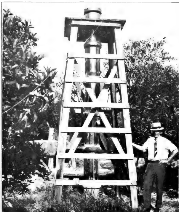
FIG. 1.—RELIEF STANDPIPE AT CONNECTION OF IRON DISCHARGE PIPE AND TERRA-COTTA DISTRIBUTING LINES, IN ORANGE GROVE, PALATKA, FLA.
