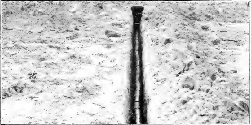
FIG. 1.—SUBIRRIGATION LATERAL TILE LAID IN TRENCH BEFORE JOINTS ARE COVERED.
