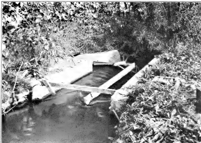
FIG. 1.—COMMON TYPE OF DIVISION BOX IN WHICH THE DIVIDING BOARD IS MOVABLE AND IS HELD IN PLACE BY A CHAIN HOOKED OVER NAILS IN A CROSS PIECE.
