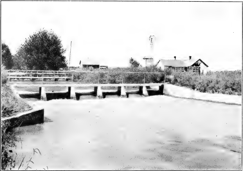
FIG. 1.—CHECK IN THE LARIMER AND WELD CANAL.
