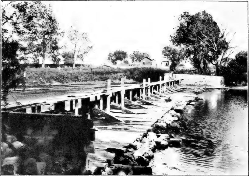
FIG. 1.—DIVERSION DAM OF THE GREELEY CANAL NO. 2.
