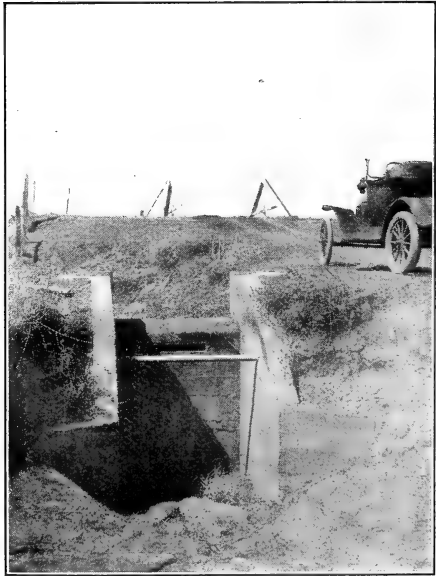
FIG. 2.—WEIR AND DROP AT THE HEAD OF THE CULVER-BARTELS LATERAL OF THE LARIMER COUNTY CANAL.
