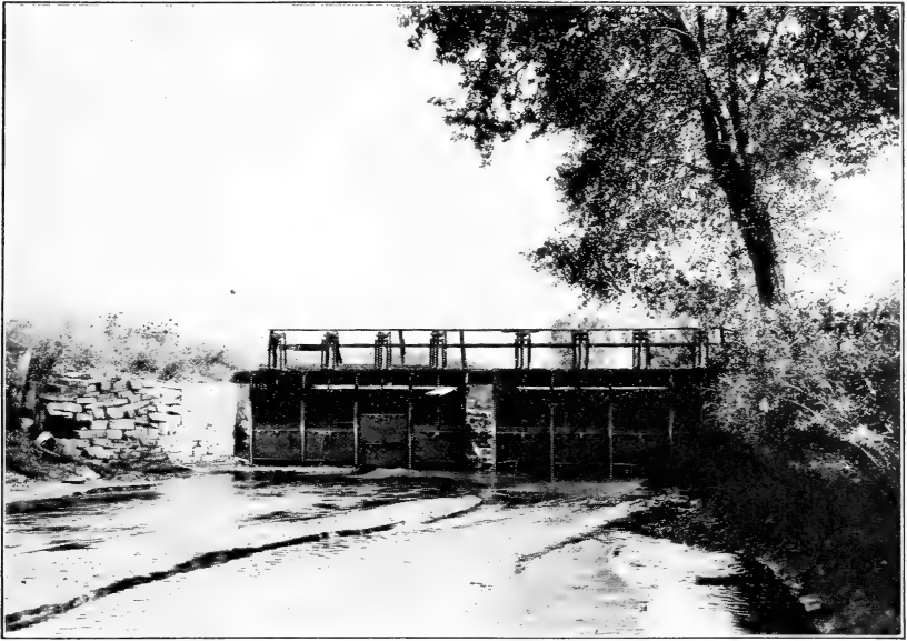
FIG. 1.—HEADGATE OF THE GREELEY CANAL NO. 2.
