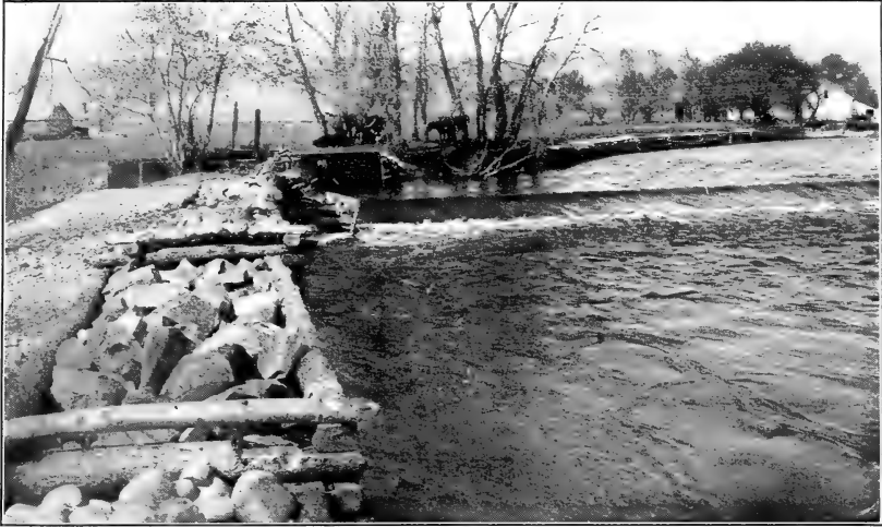
FIG. 1.—ROCK-FILLED CRIBS USED AS RIVER PROTECTION AT THE HEAD OF THE ARTHUR DITCH.
