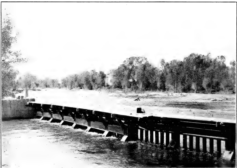
FIG. 2.—DRIFT GUARD AT HEAD OF LARIMER AND WELD CANAL.
