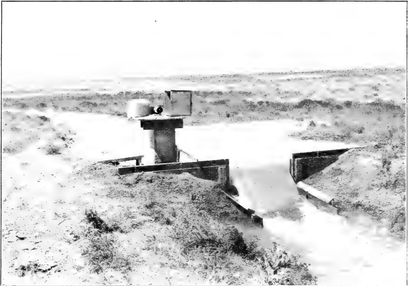
FIG. 1.—WEIR ON THE OUTLET OF THE DEALY RESERVOIR. AVERAGE OUTFLOW.
