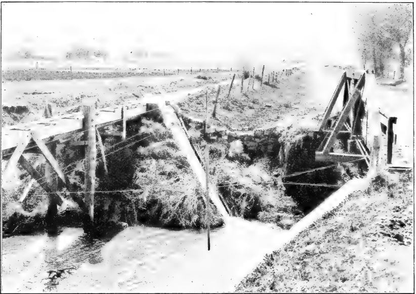
FIG. 1.—FLUME CARRYING TAIL OF LITTLE CACHE LA POUVRE DITCH OVER DRY CREEK.
