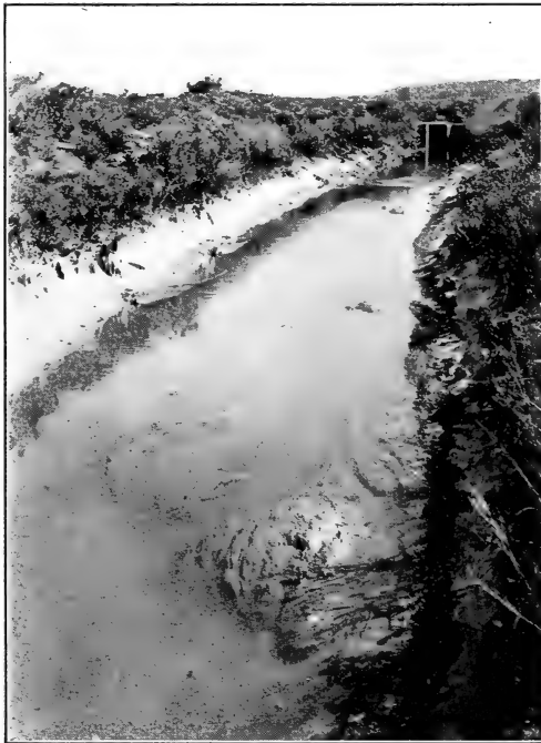
FIG. 2.—MOSS IN THE OUTLET OF THE ROCKY RIDGE RESERVOIR.
