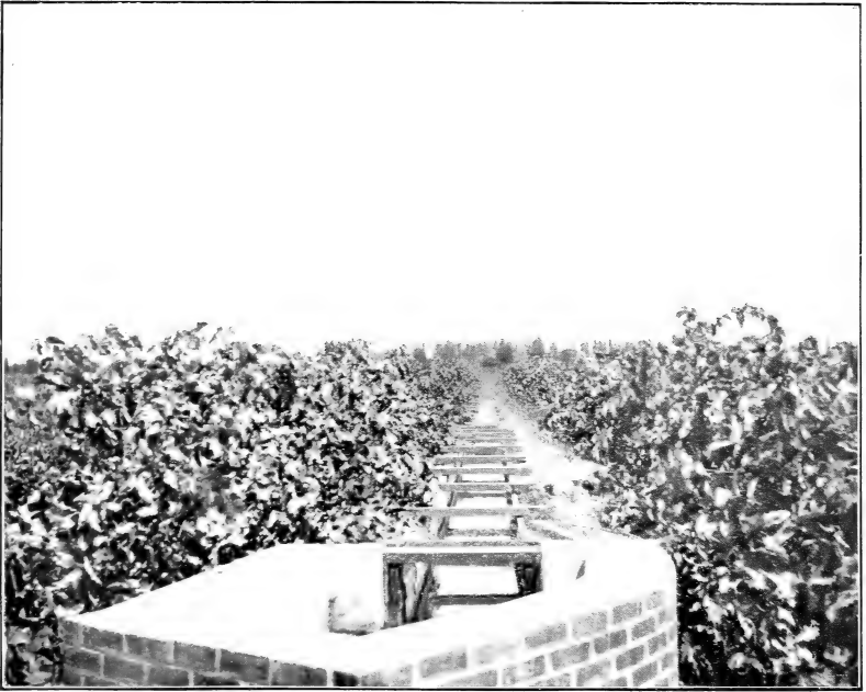
FIG. 1.—AQUEDUCT BENEATH A HIGHWAY FROM A MAIN DITCH TO FLUME SUPPLYING A VINEYARD.
