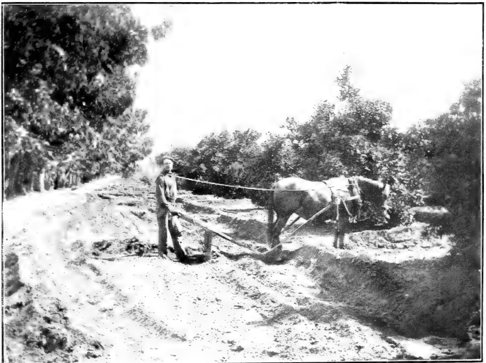
FIG. 2.—STARTING WITH THE "JUMP SCRAPER" TO CLOSE A ROW OF GAPS.
