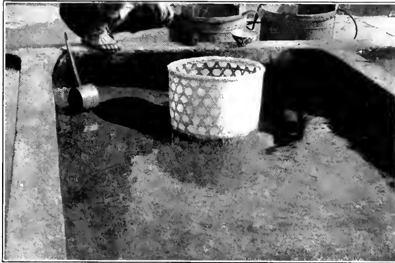
DRAWING DOWN A CONCRETE REARING POND
