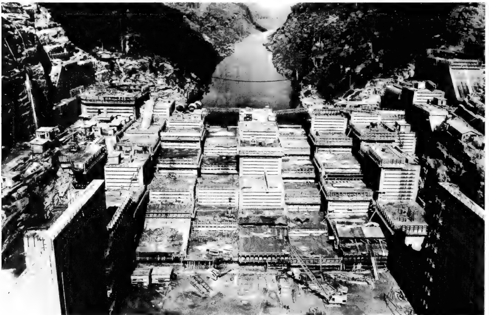
Figure 10: Warragamba Dam main wall construction.
