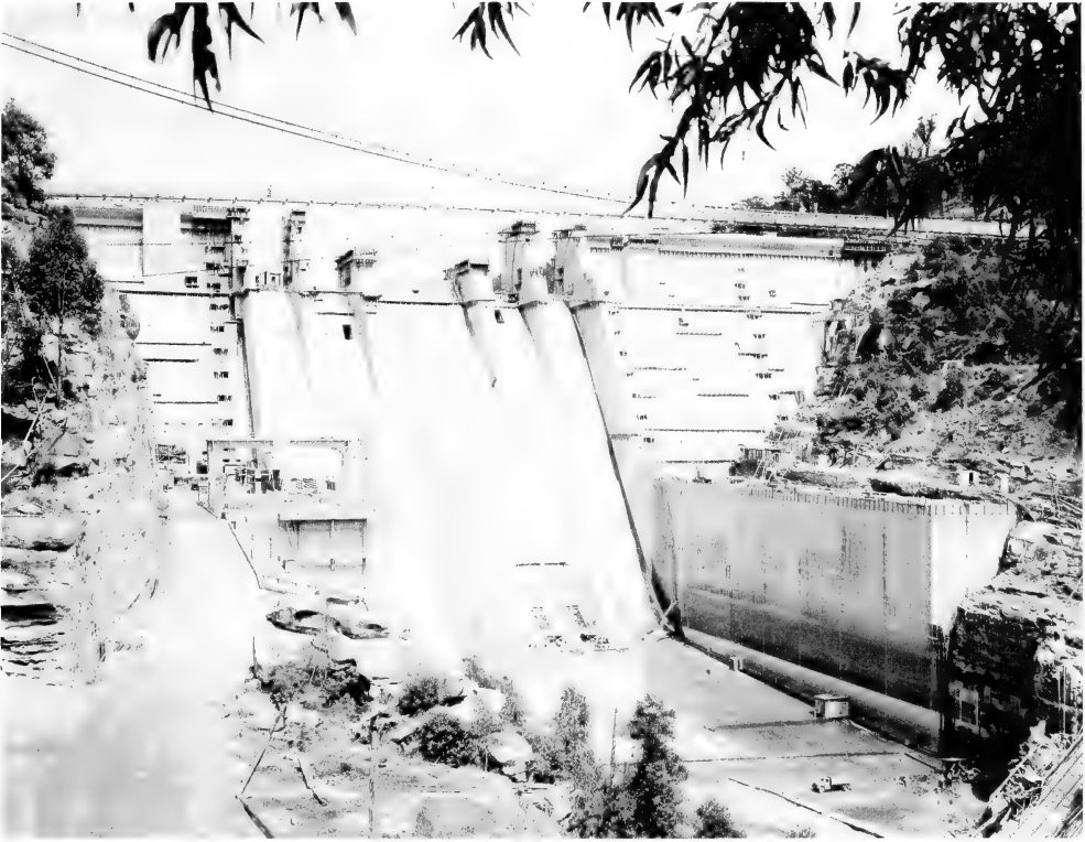
Figure 11: Warragamba Dam nears completion.
