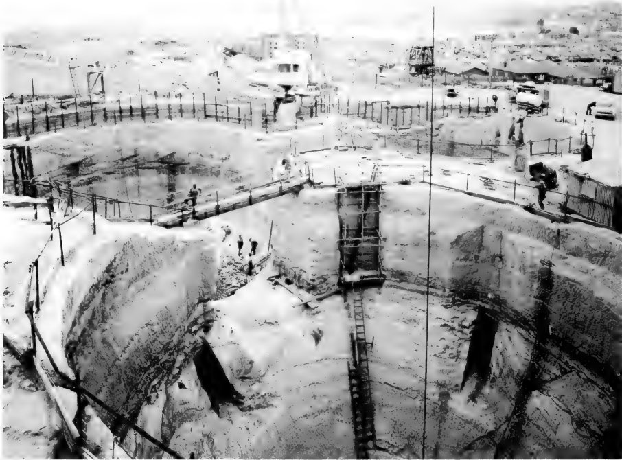
Figure 12: Bondi Sewerage Treatment Works under construction in 1984.
