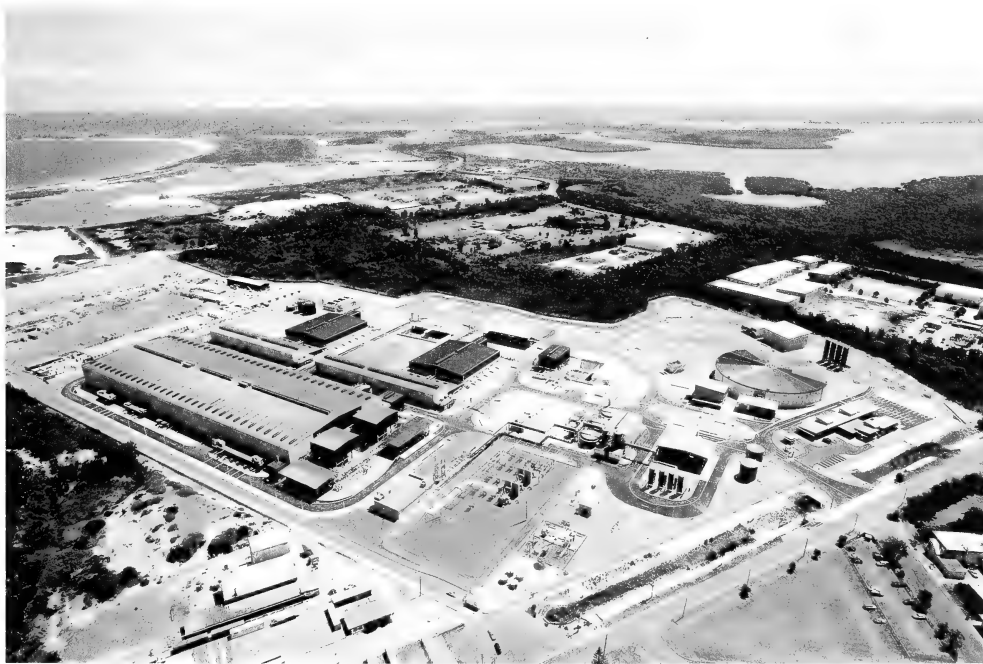
Figure 13: Desalination plant, Kurnell, 2008.
