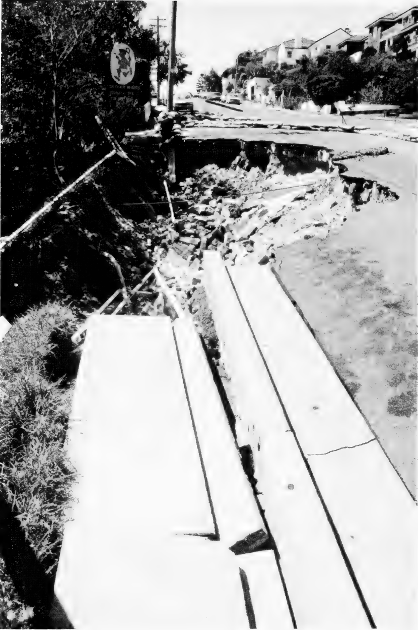
22. Heavy erosion in Hardy Street caused largely by restricted flow derived from Macleay St. (first right) which has a steep cliff at its eastern end.
