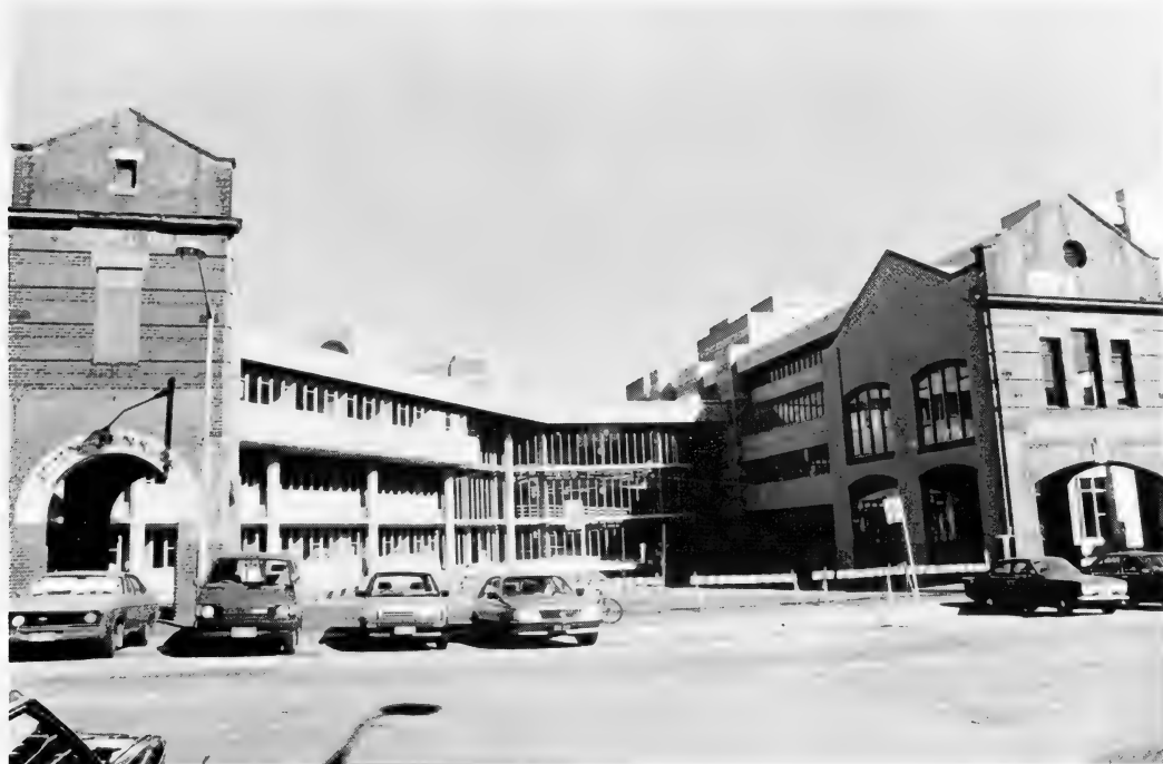
Figure 8. Philip Cox, New South Wales Institute of Technology extension, incorporating the old Fruit and Flower Markets, Haymarket.
