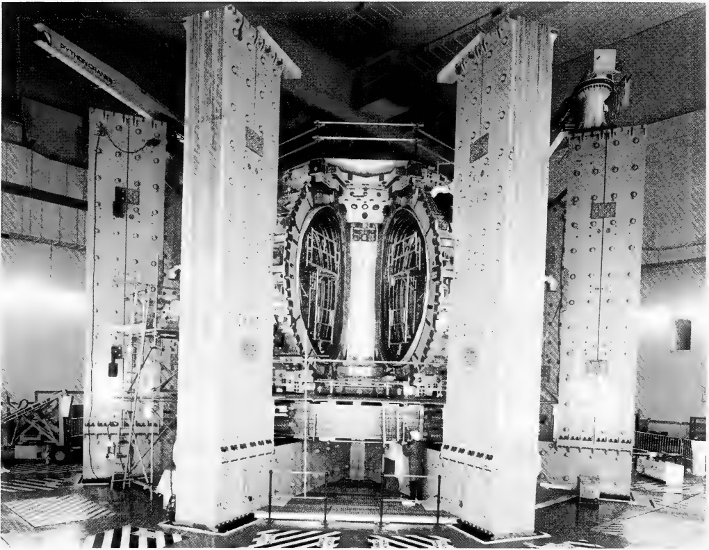
Figure 10. The Joint European Torus, JET, during construction. Four of the eight outer limbs of the transformer core await the top horizontals connecting them to the central core. The D-shaped minor cross-section of the toroidal vacuum vessel is seen in the gap left for the final octant, still to be fitted and welded into place.
