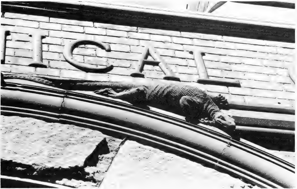
Figure 6. Detail of carving over main door, Sydney Technical College.
