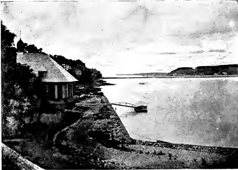
COLD SPRING HARBOR, WITH A VIEW OF THE EAST END OF THE LABORATORY.
