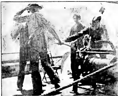
DREDGING ON "POURTALES PLATEAU."
